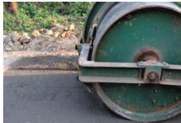
Fig.3: Rolling of cement-sand filled into cells
