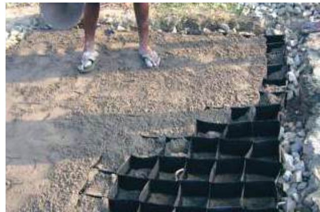
Fig.2: Cement-sand mixture being filled into cell the cells at OMC
