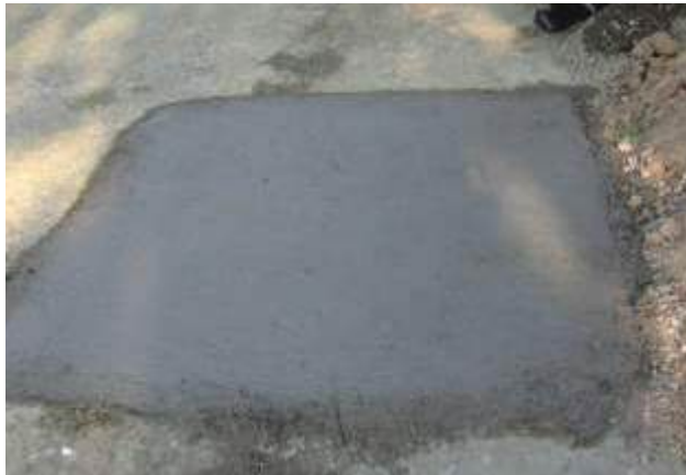
Fig.4: A view of finished surface
