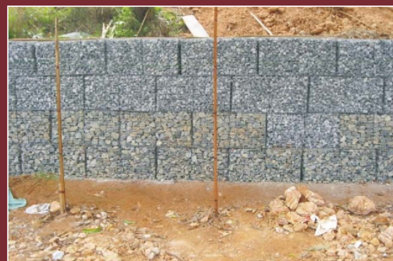
Fig. 8 Front view of the completed gabion facing retaining wall.
