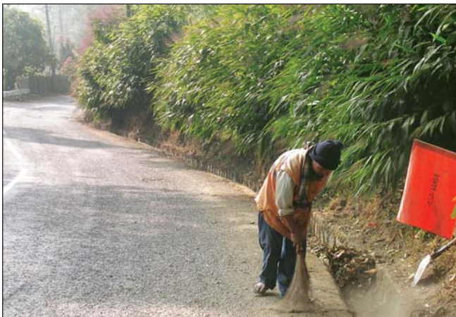
Fig 3. On Road Routine Maintenance
