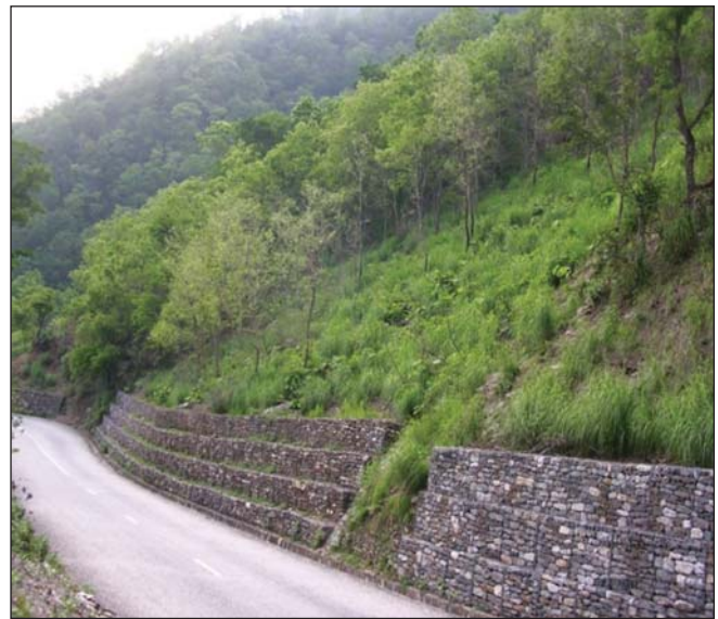
Fig 4. Road side Bio-engineering
