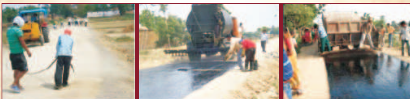
FIGURE 2. Otta Seal Laying Process cleaning, bitumen spray and chips spreading.
