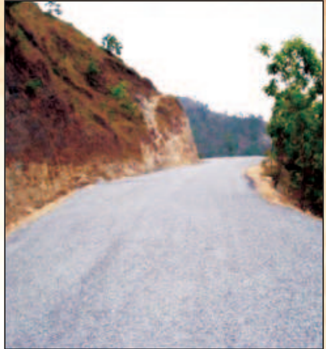
FIGURE 1. Freshly-laid Otta Seal
