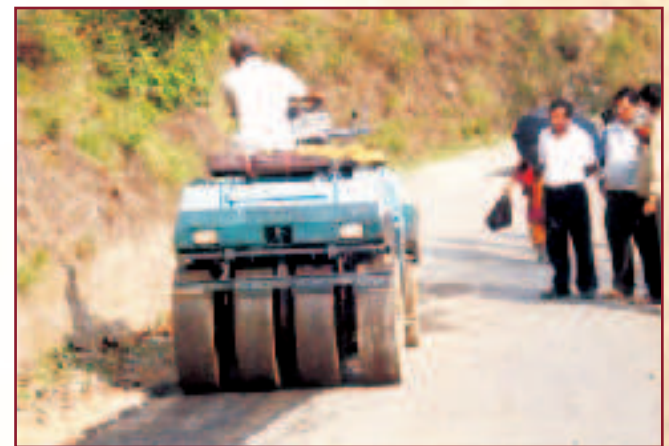
FIGURE 6. Otta Seal maintenance
