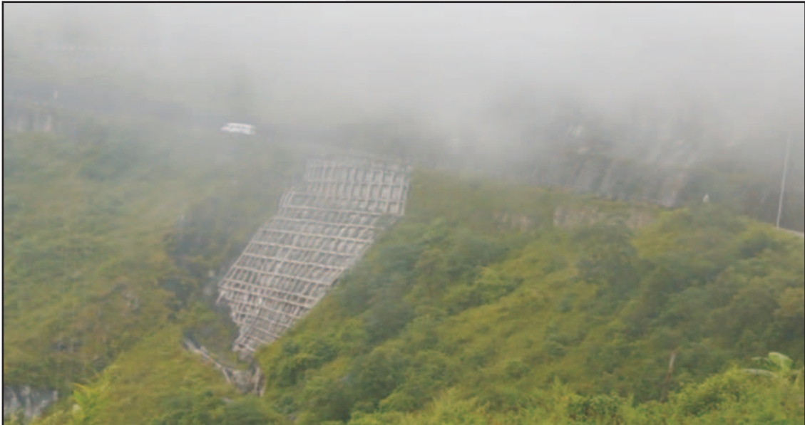
e) Rock bolting/Stabilization of slopes/fractured rocks by construction of RCC bands bolted with high tension steel cables
