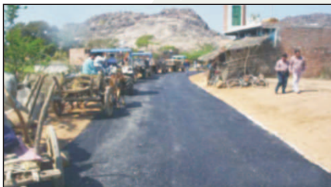
Photograph 1- Habitation along PMGSY Roads creates Hazards to Road Safety
