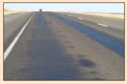
Spread heated chippings: On areas with excessive bleeding, spreading heated chippings of nominal size 6 to 10 mm is more effective due to the amount of binder. The chippings can be heated in a tray over open fire and rolled into the bitumen for proper embedment.
