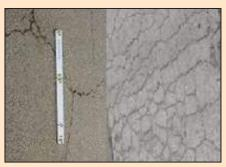
Sealing of fine cracks < 3 mm wide (frequent and closely spaced cracks within a limited area), can be carried out by applying a fog seal to the damaged surface, consisting of a light application of low viscosity slow setting emulsion.
