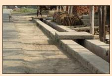
This activity includes provision of construction materials and repair of damaged drain lining to its intended shape and specification as directed by the Engineer. The masonry work shall be cured for at least 4 days.
