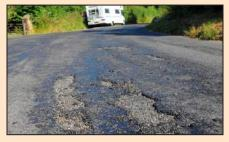
**On-carriageway works** relate to road pavement and surface repairs. This work mainly consists of maintaining a good running surface on the road, free from any obstructions and damage and with the necessary camber or cross-fall to secure proper surface drainage.
