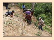
The activity includes furnishing and planting turf and sods, achieving a healthy stable covering of grass which will maintain its growth in any weather. This is to prevent erosion of the material in which it is planted and stability of side slopes and embankments.
