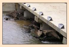
This activity includes clearing of silt, debris and litter around the structure, its abutments and piers and for a minimum distance of 25 metres both up stream and down stream thereby allowing water to flow freely and unhindered. All matter should be removed clear of the river and the drainage system to prevent it from being washed back into the waterway.
