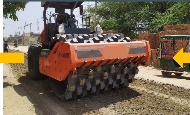
Compacting using heavy duty 15-20 Ton Padfoot Roller Hamm 139i D
