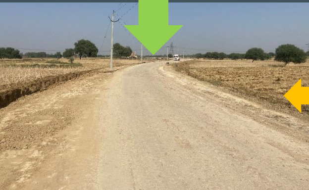
Stabilized Base using FDR technology
