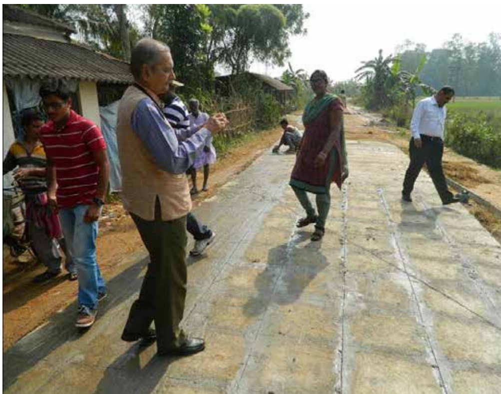
Whitetopping with short panels of 0.5 m x 0.5 m
