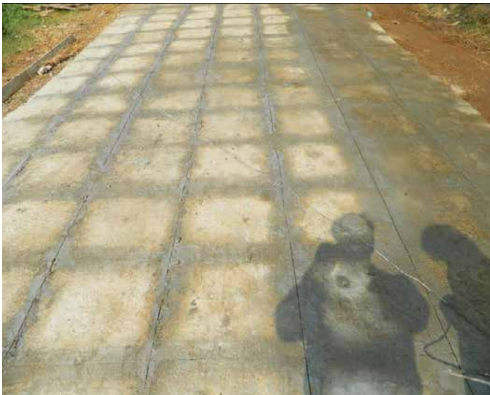
Whitetopping with short panels of 0.5 m x 0.5 m
