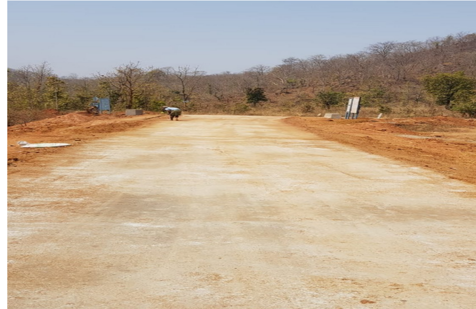
Stabilized Surface after curing
