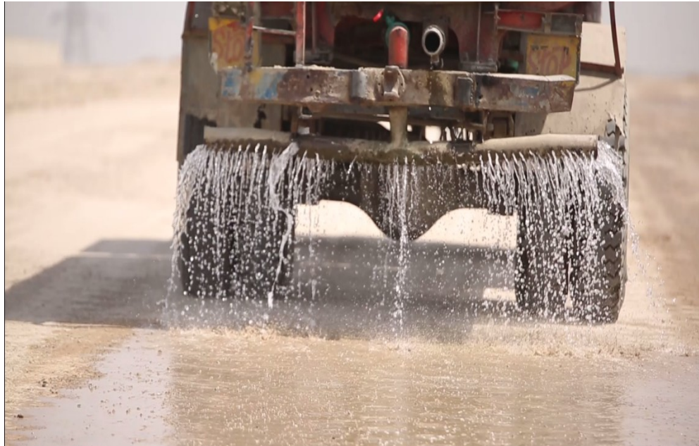
Curing of the stabilised layers
