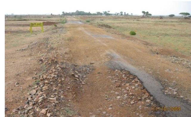
Extensively Worn out Pavement
