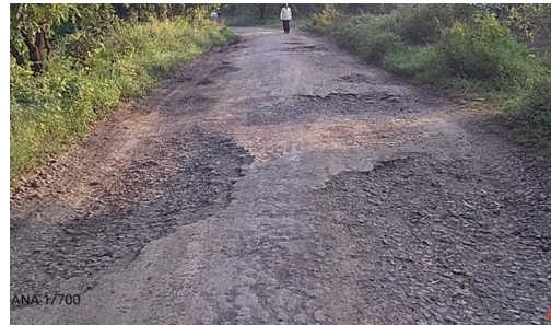
Extensively Worn out Pavement
