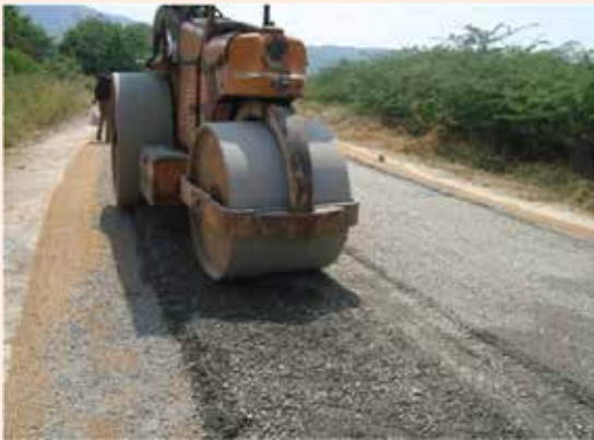
(f) Laying & compaction of GSB
