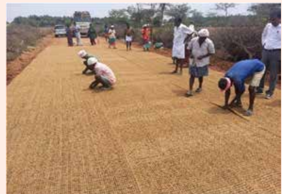
(e) Pinning the edges of coir geotextiles
