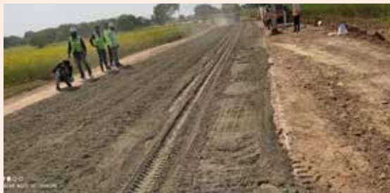
Spreading of Cement and Additive
