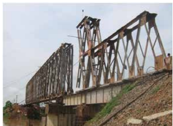
Figure 5: Elevation - Patent Information, Elevation on Callender-Hamilton Bridge
