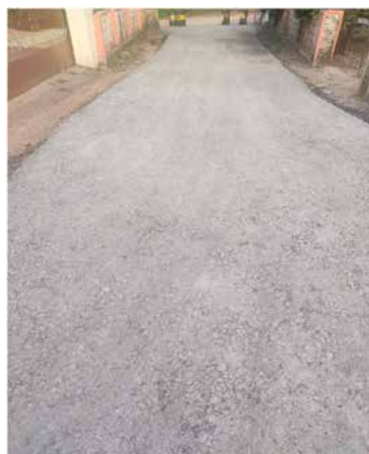
Figure 10: ETB after 24 hours curing
