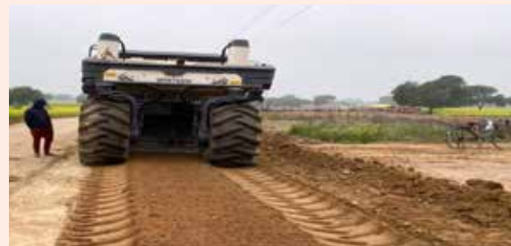
Recycling of existing crust
