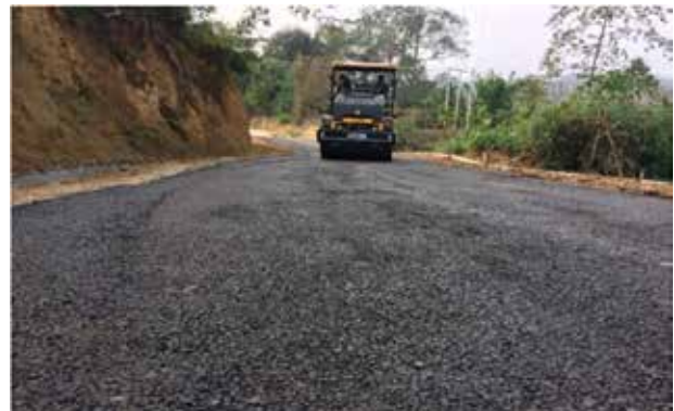
Compaction of OGPC layer
