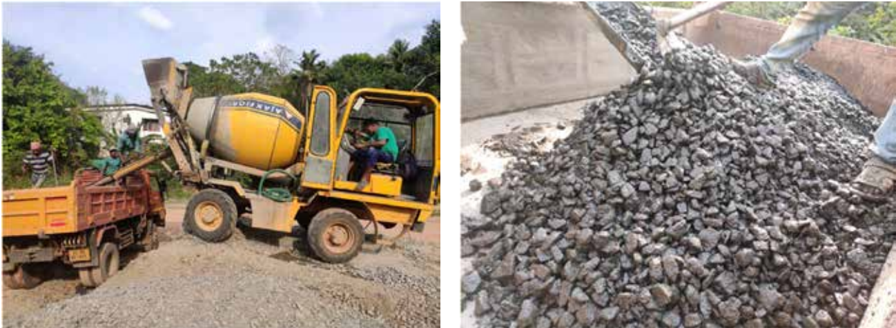
Figure 4: Preparation of ETB using conventional concrete drum mixer
