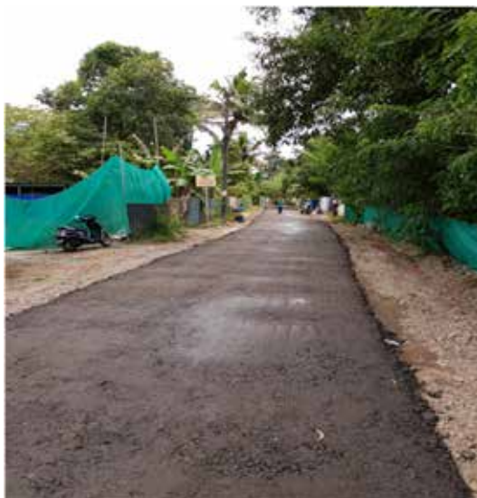
Figure 7: Compacted ETB surface
