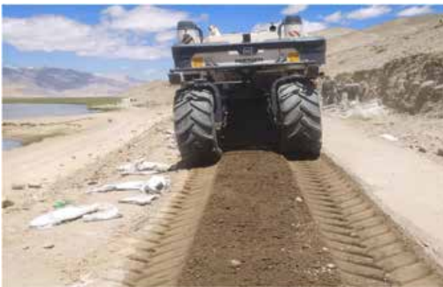
Figure 5: Rolling of Cold Mix Bituminous Macadam layer
