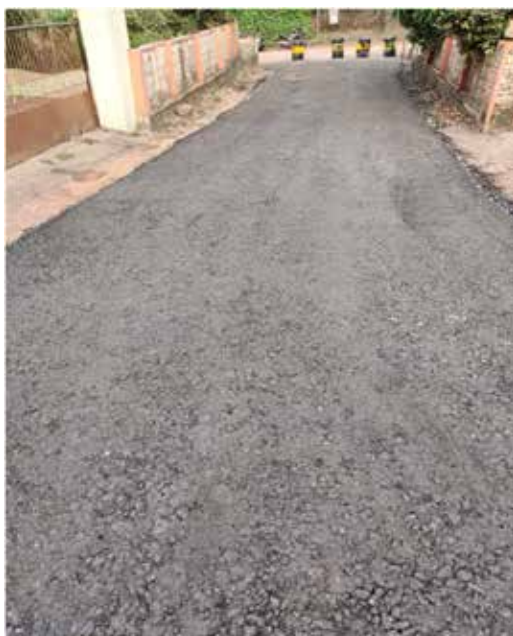
Figure 9: ETB after construction
