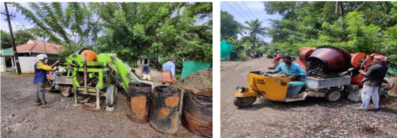
Figure 4: Preparation of ETB using conventional concrete drum mixer
