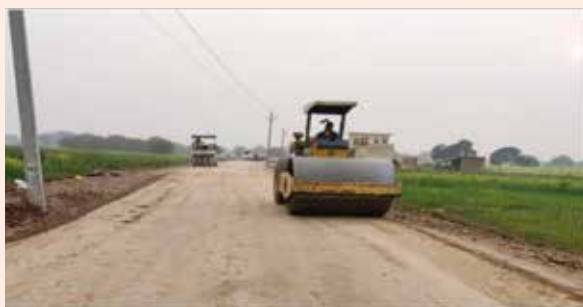
Compaction by compactor and PTR
