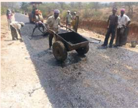
(h) Laying of premix concrete
