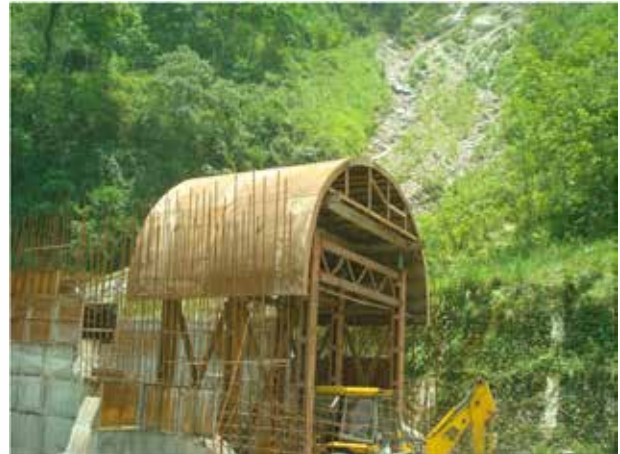
Figure 8: Fabricated Gantry for casting of curved roof
