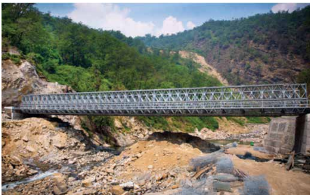
Figure 3: Permanent Modular Bridge – Erected at Sonprayag, in Uttarakhand after the 2013 Floods
