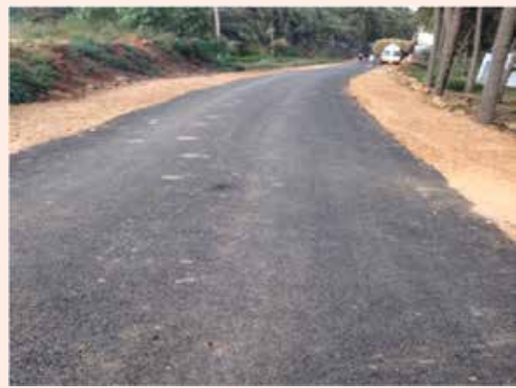
(i) Finished road
