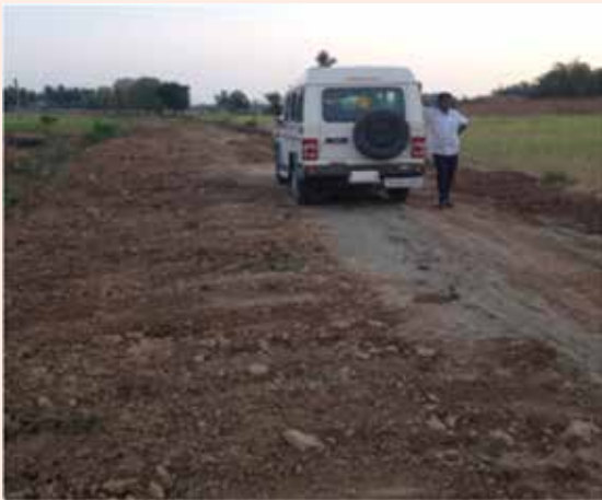
(a) Preparation of subgrade
