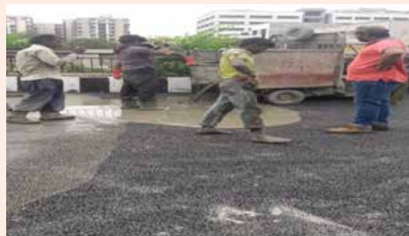
Grouting in bituminous layer (Stage 2)
