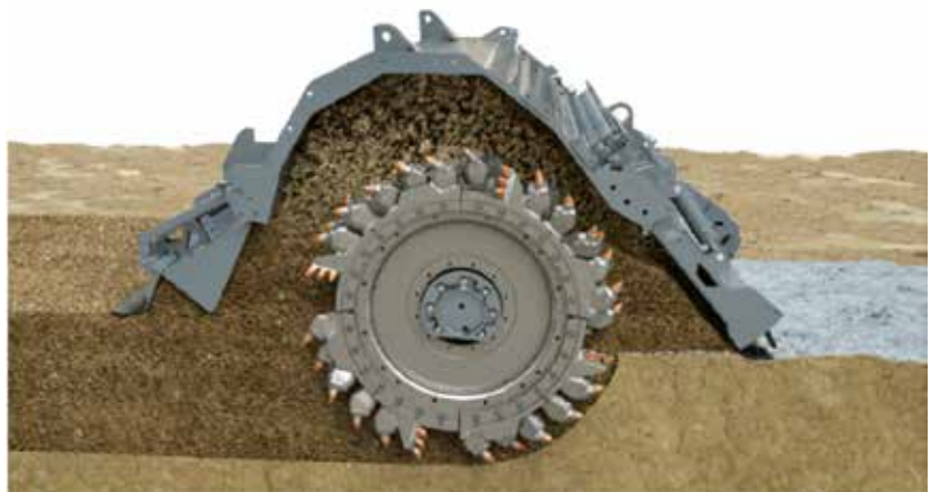
Figure 2: Mixing during construction of CTB layer
