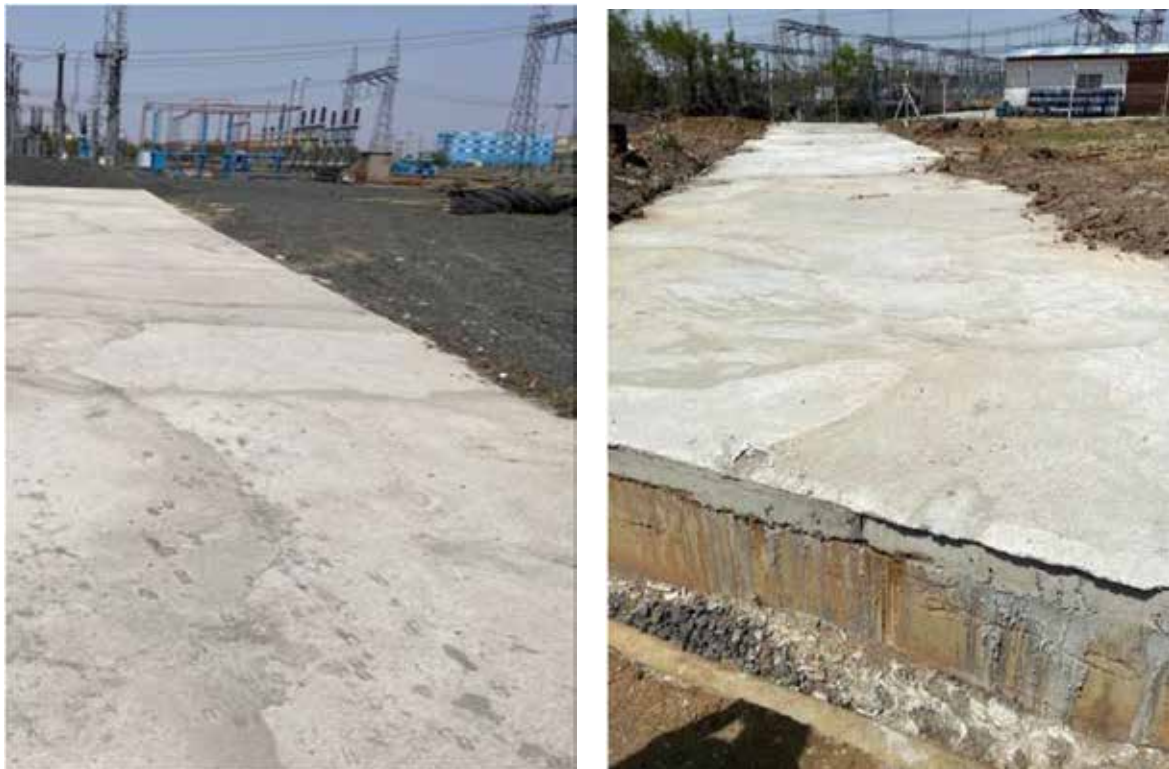
Figure 1: Constructed Road patch at NTPC Mouda
