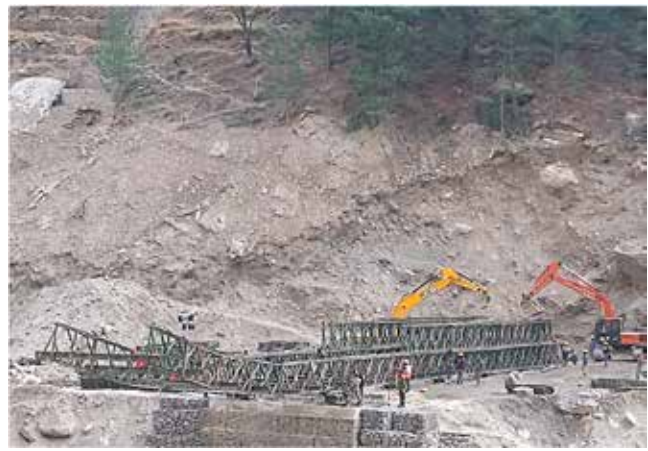
Figure 10: View of completed 200 feet span Bailey bridge
