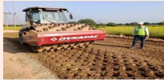
Compaction by Padfoot Roller
