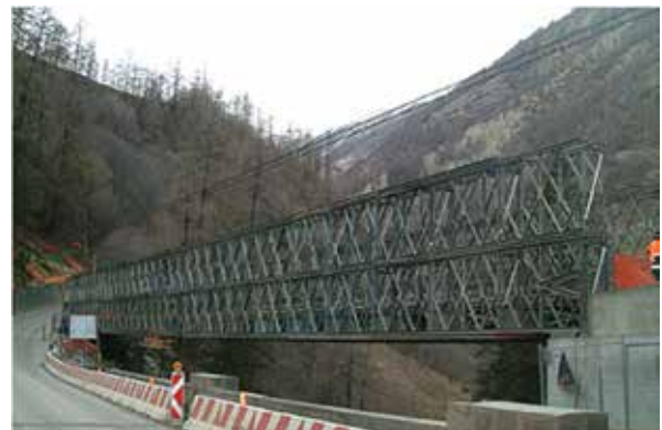
Figure 11: Quadricon Modular Bridge across Dhaman Khad
