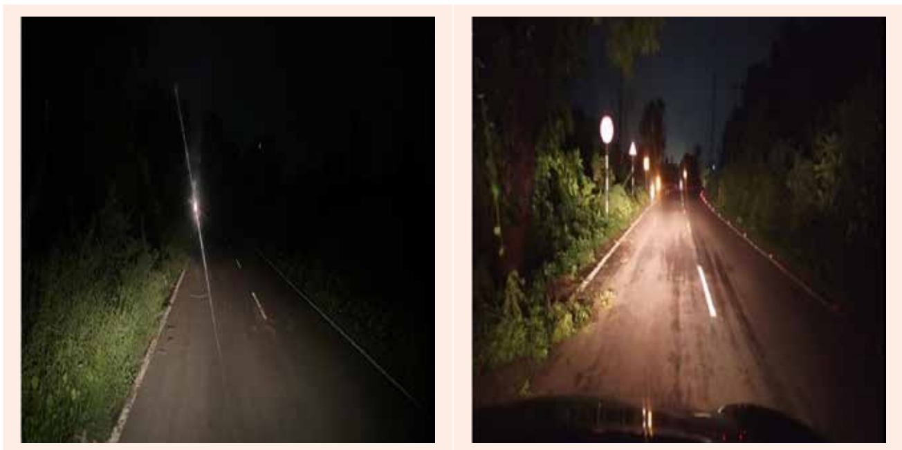
Figure 3: Before and After Condition of Roads with the implementation of Road Signage and RPMs
