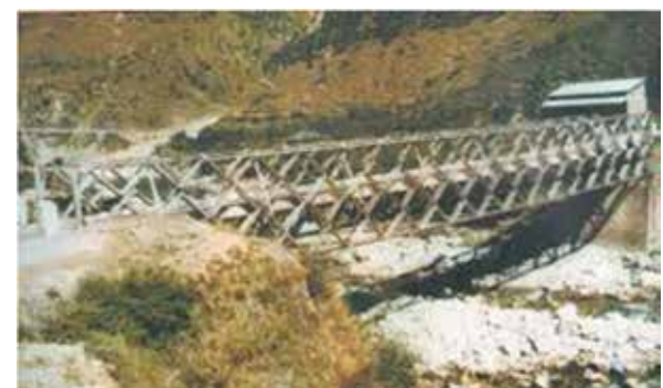
Figure 11: Quadricon Modular Bridge across Dhaman Khad
