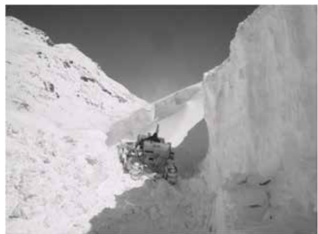
Figure 2: Deployment of dozer for Snow clearance
