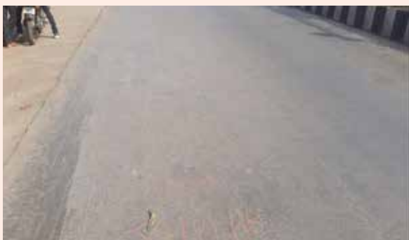
Finished surface of CGBM (Stage 3) in June 2017
