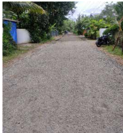
Figure 8: Compacted WMM surface
