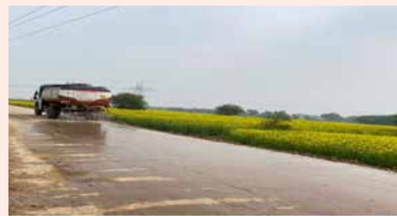
Water curing of FDR Base
