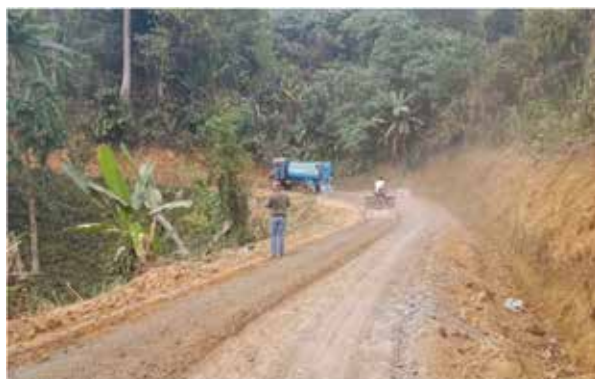
Soil-cement stabilization process in progress
