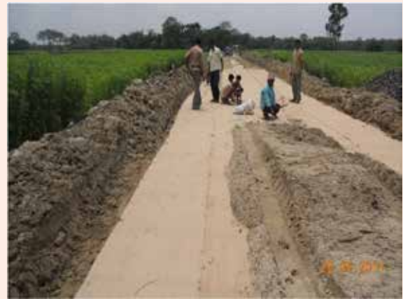
Laying of JGT followed by Spreading of Sand
