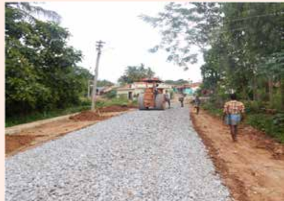
(g) Laying & compaction of base layer
