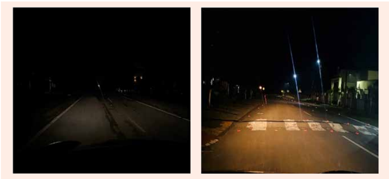
(b) Improved edge line delineation after RPM installation at Maroli Site
