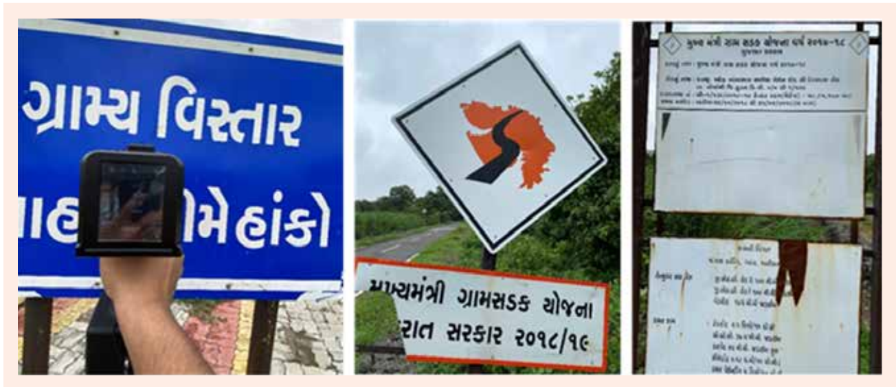
Figure 2: The Traffic Sign Condition Survey and Testing
