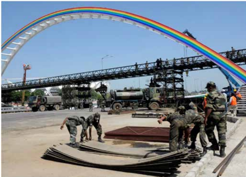
Figure 2: Emergency Modular Bridge – Erected in 5 days before CWG 2010
