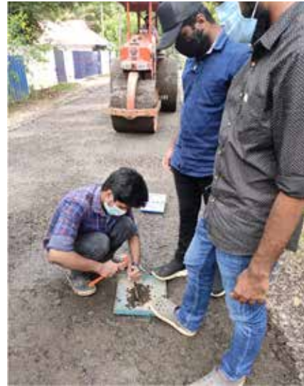
Figure 6: Sand replacement test on ETB
