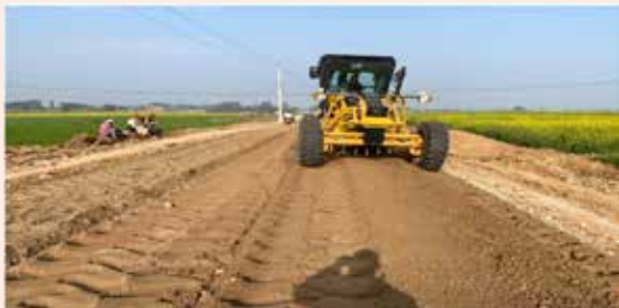
Grading of FDR material
