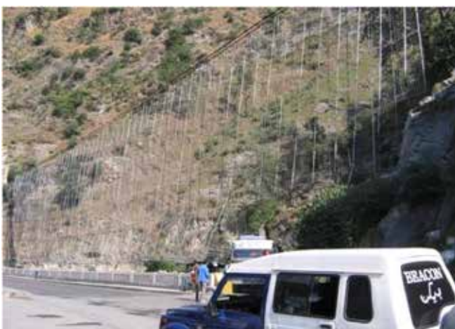
Figure 1: Safety net to arrest shooting boulders
