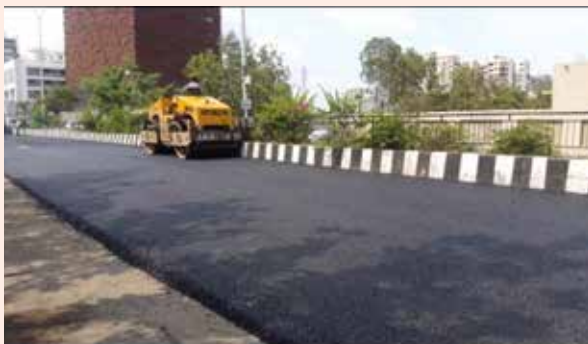
Paved High Voids bituminous layer at site (Stage 1)
