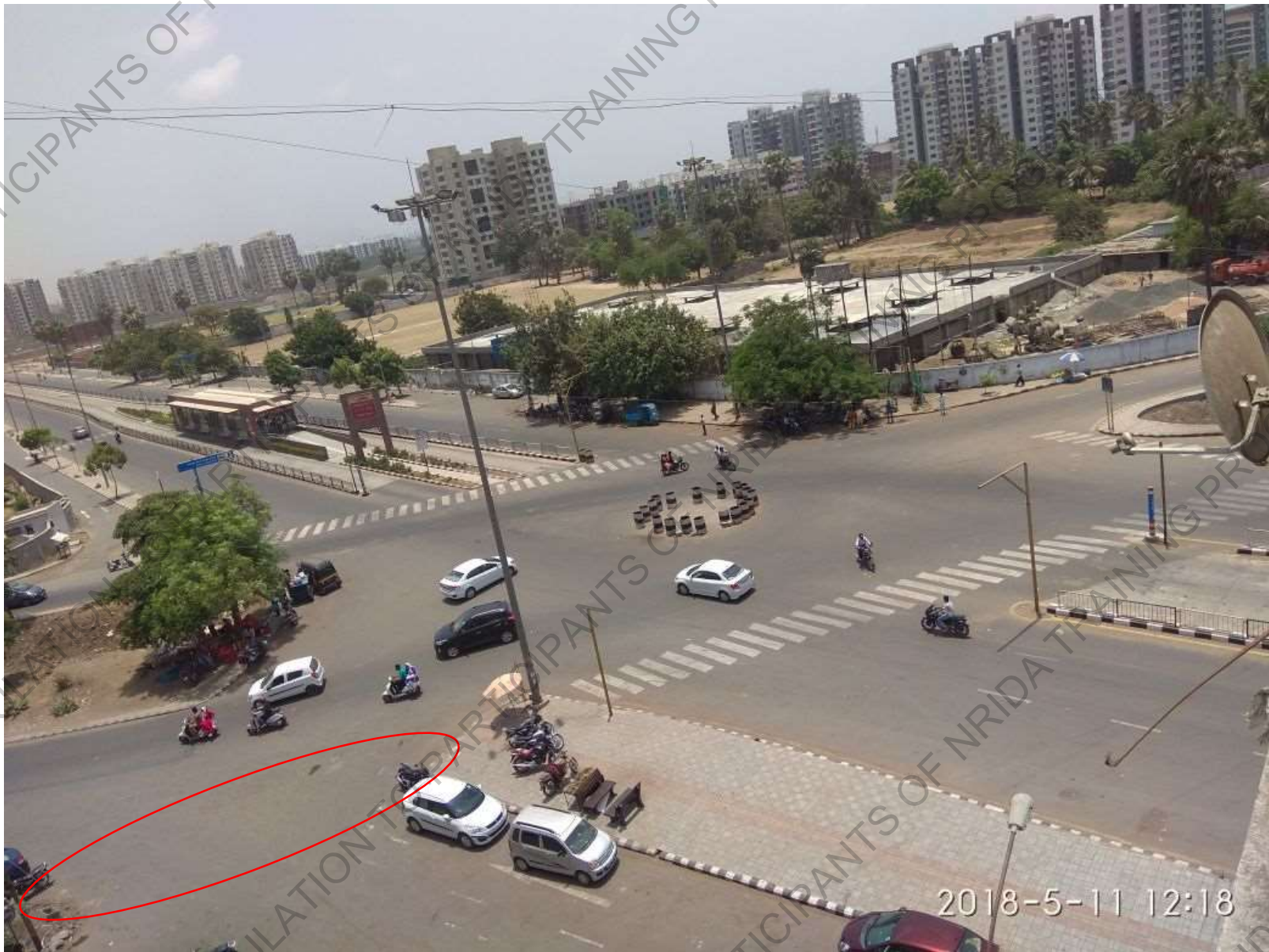
Crosswalk marking is discontinued in between, but it should be provided till the end, kerb-kerb or shoulder-shoulder
