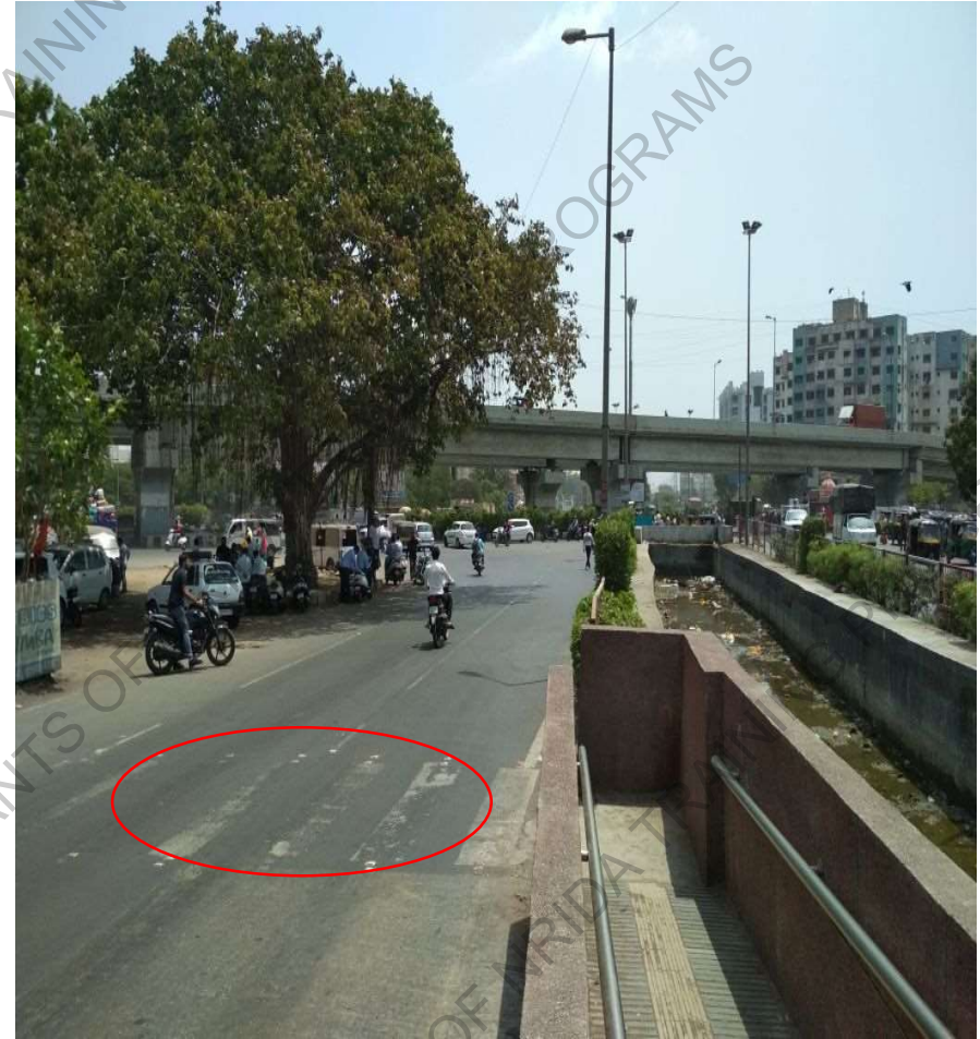
Overlaying road markings and performing timely scheduled maintenance
