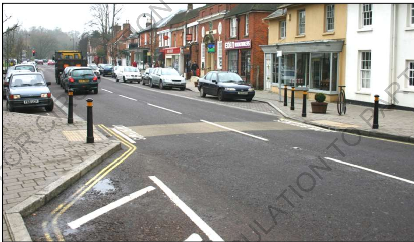
Extending the footpath at a crossing
