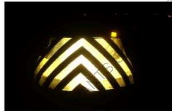
Night Visibility of Bullnose after applying AFP Sheeting
