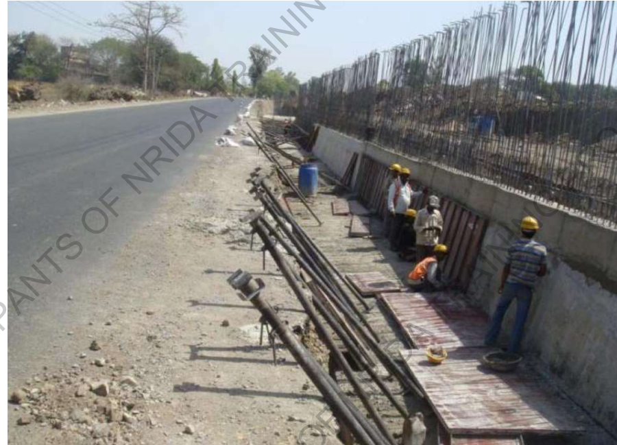
Unprotected operations & workers in work zone
