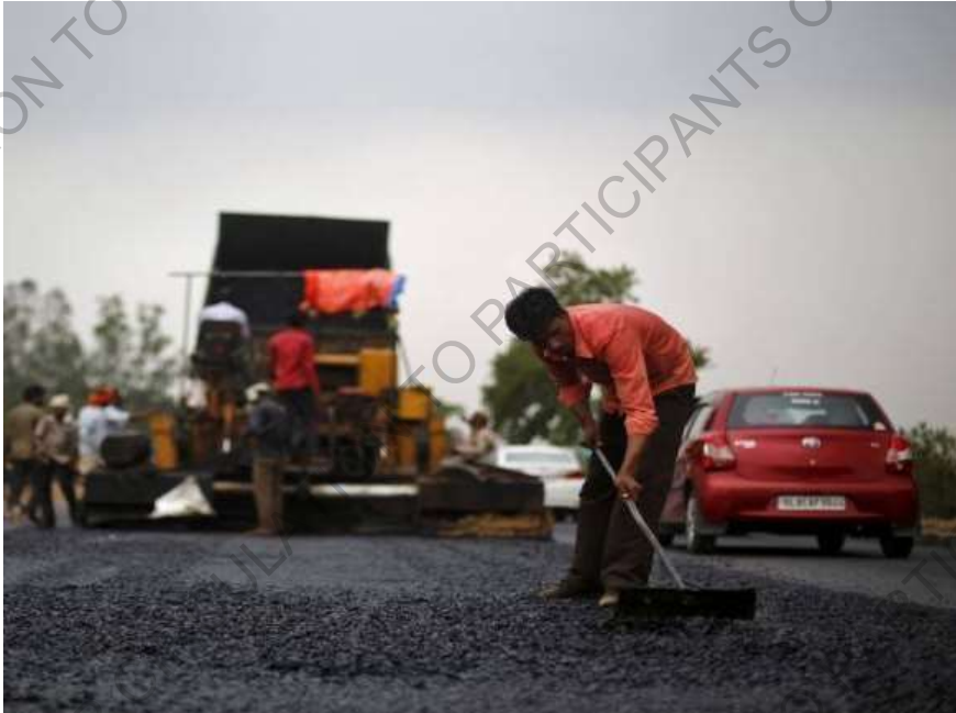
Unprotected operations & workers in work zone
