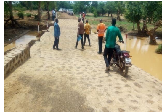
Images of construction of crossing structures on a rural road
