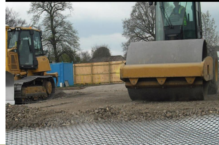
COMPACTION OF BASE WITH GEOCELLS
