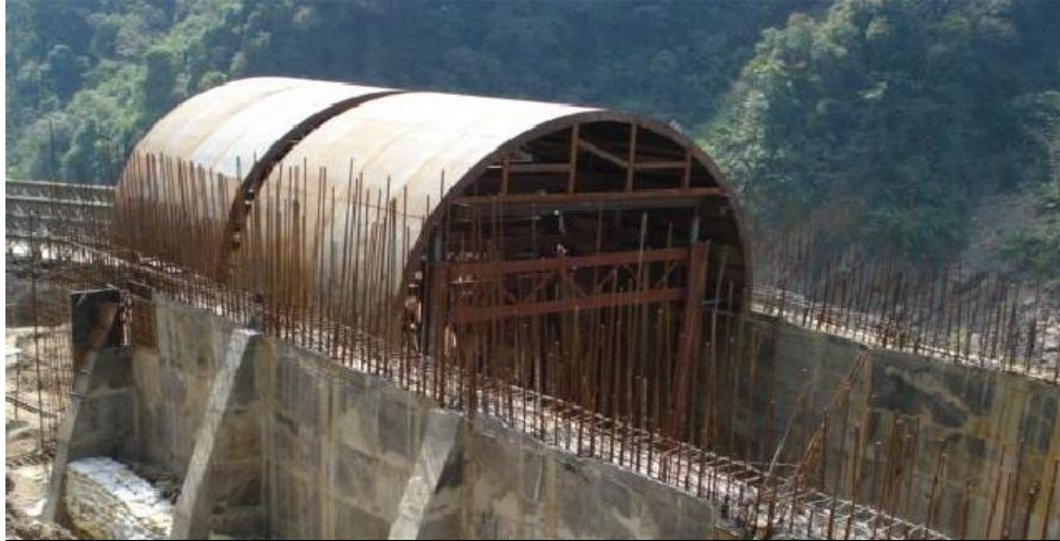
ERECTED GANTRY FOR CONCRETING OF SEMI CIRCULAR ROOF
