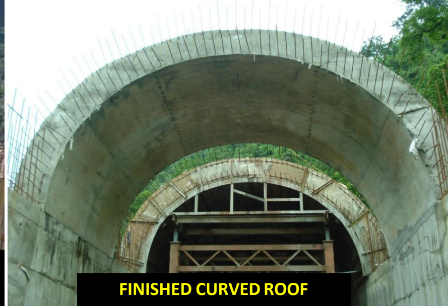
ERECTED GANTRY FOR CONCRETING OF SEMI CIRCULAR ROOF
