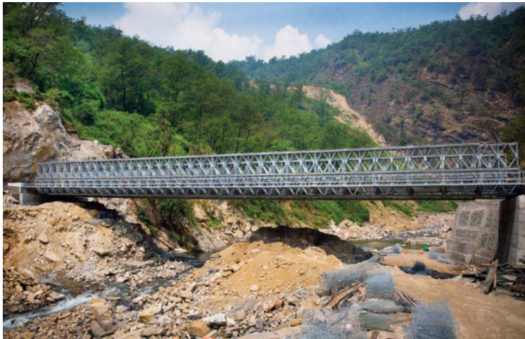
Permanent Bridge Sonprayag Bridge-Uttarakhand (Post-Disaster 2013 Floods)
