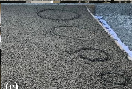
Preparation of Infiltration Rings for Field Placement of PC Test Section
