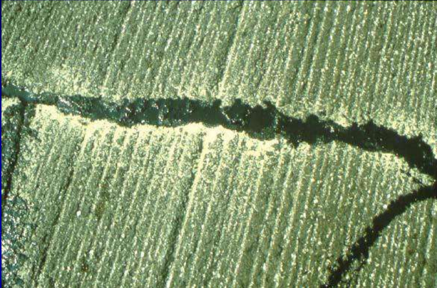
Sealed Crack
