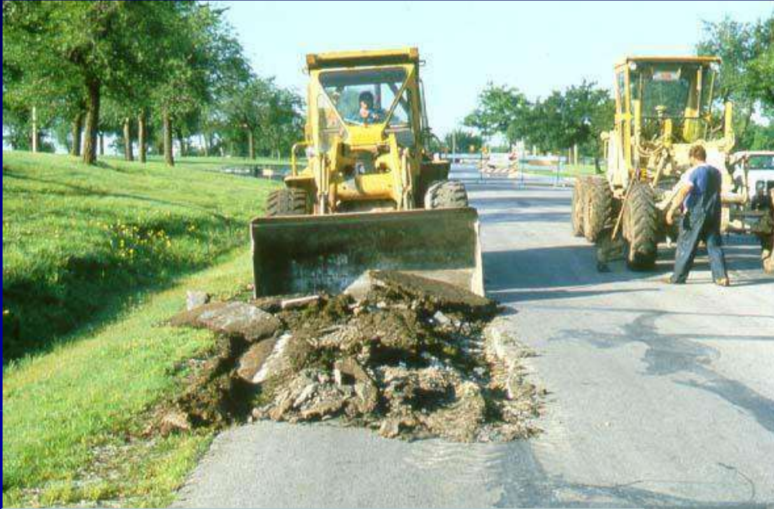
Remove Rutt/Fatigue Section and Repair Subgrade/Base
