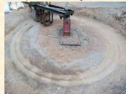
Preparation of sub-base after test
