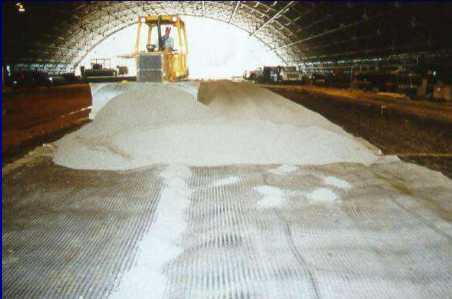
Aggregate Placed In Center and Spread To Shoulders Over Geosynthetics
