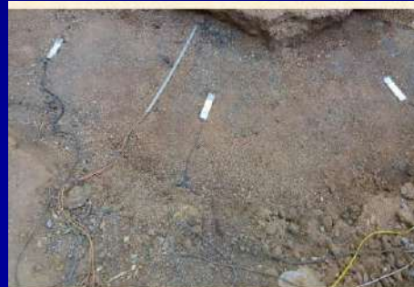
Preparation of sub-base and installation of sensor
