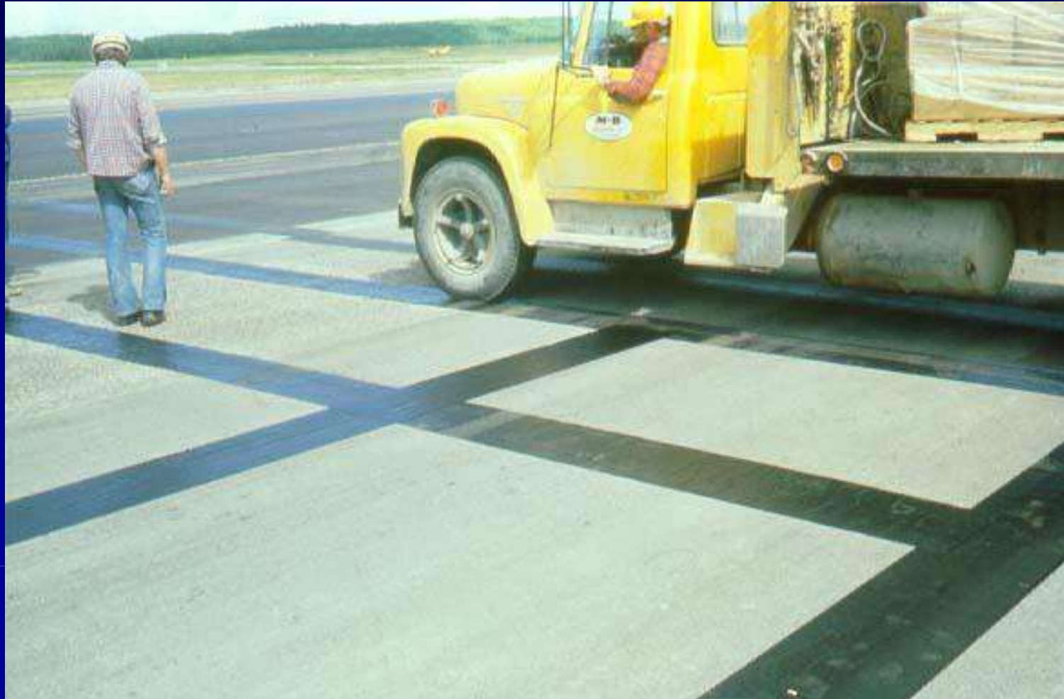
Seat Interlayer Material with Modern Equipment
