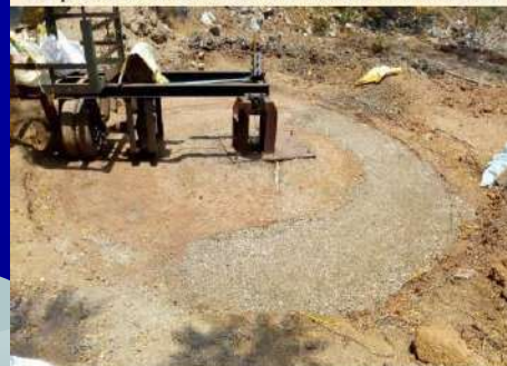
Preparation of sub-base before test
