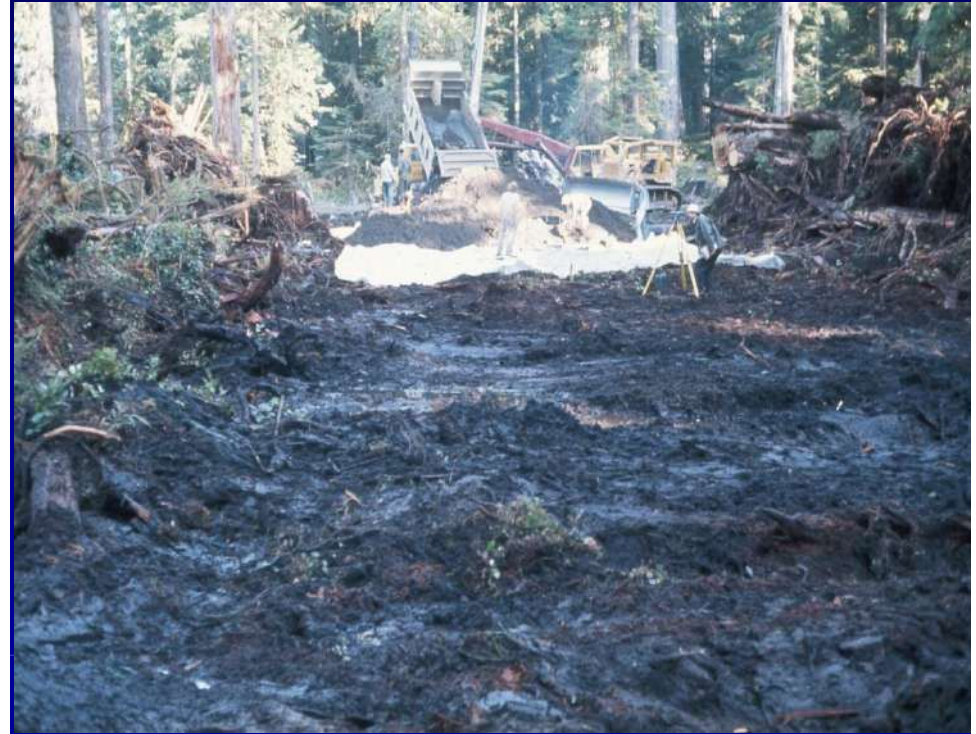
C. Back dump aggregate onto the previously placed aggregate. Do not drive on the geotextile. Maintain 6 to 12 inches (150 to 300 mm) cover between the truck tires and geotextile.
