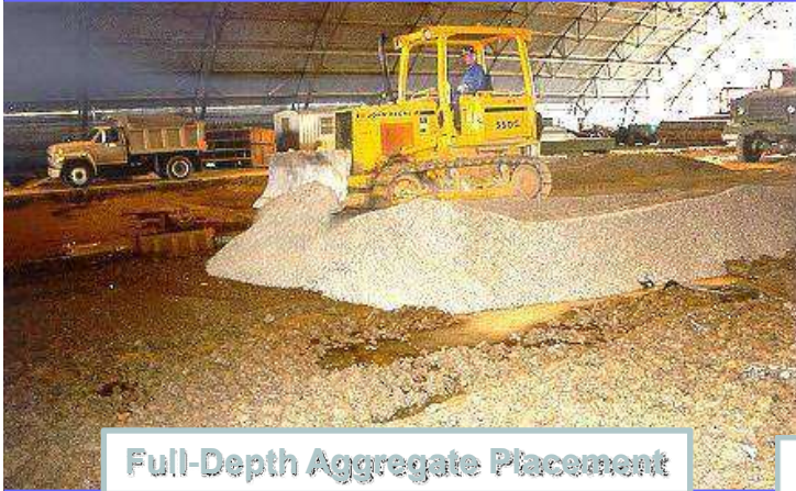
Spread Aggregate To Shoulders
