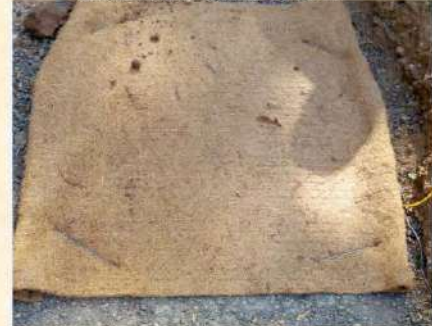
Installation of coir geotextile
