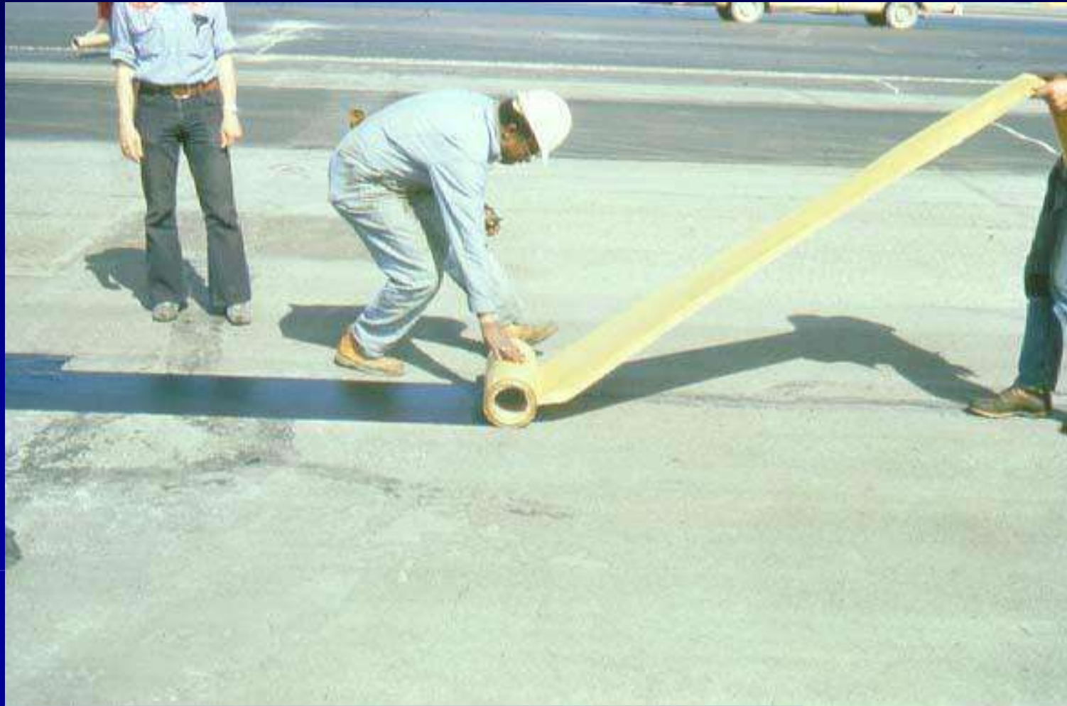
Band-Aid Interlayer for PCC or Reflective Cracking
