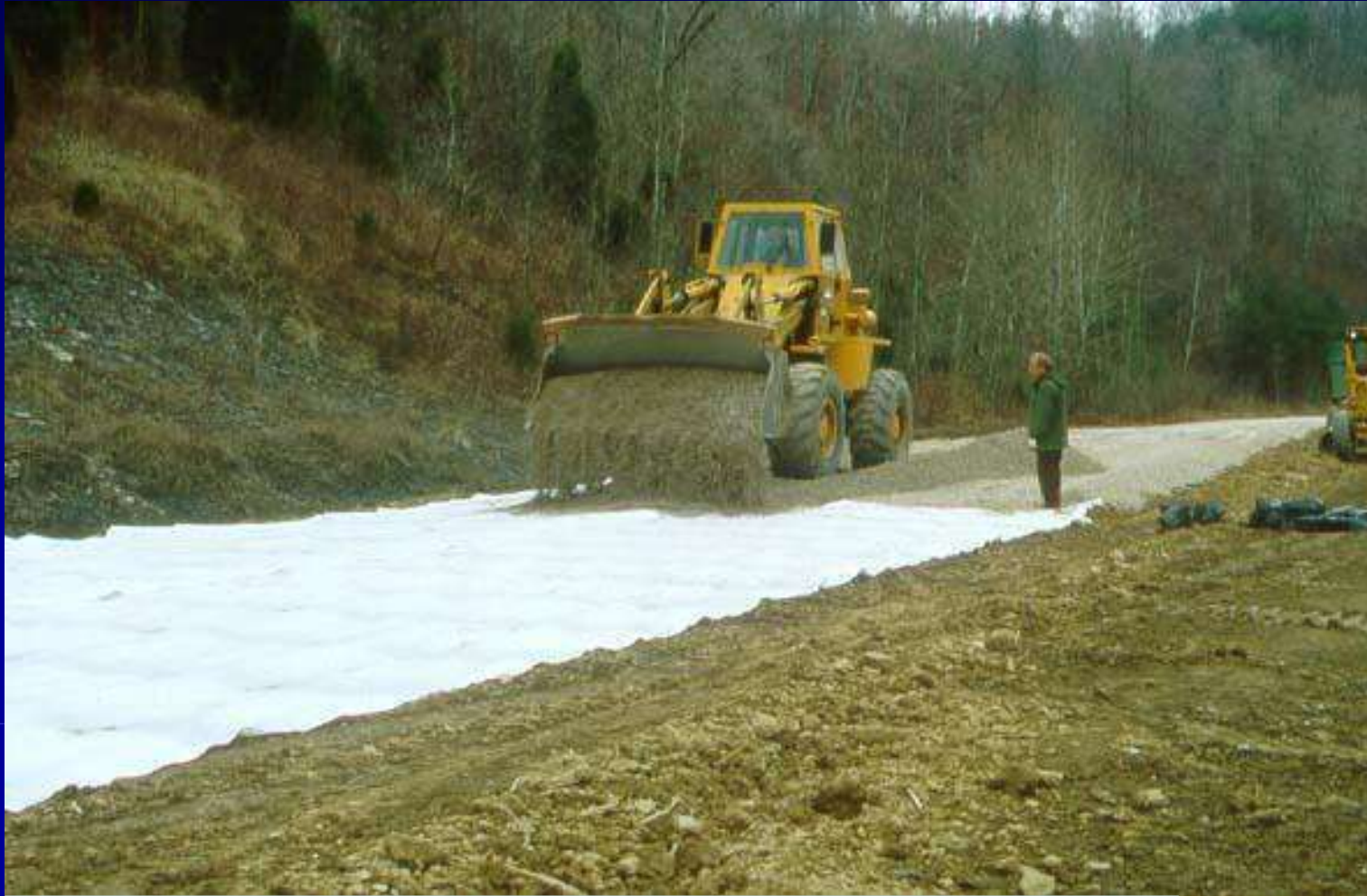
Aggregate Placement – Avoid Thin Lifts (Probably Too Thin Here)
