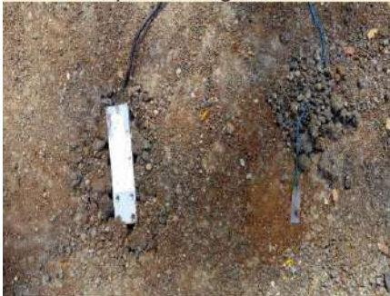
Installation of load cell and strain gauge
