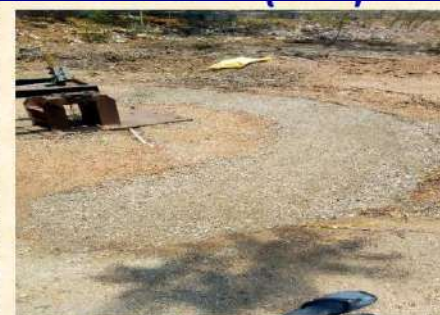
Compacted sub-base with gravel soil
