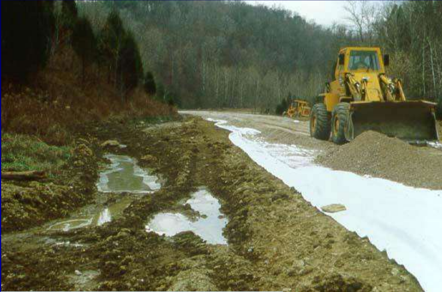
Spread Aggregate From Center to Shoulders
