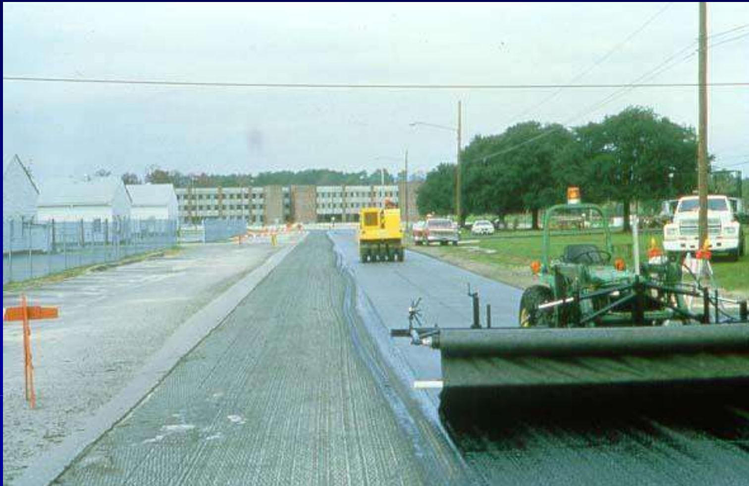
Seat Fabric With Pneumatic Roller to Ensure Intimate Contact With Surface
