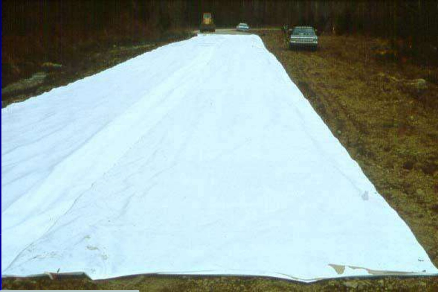
Geotextile Placement
