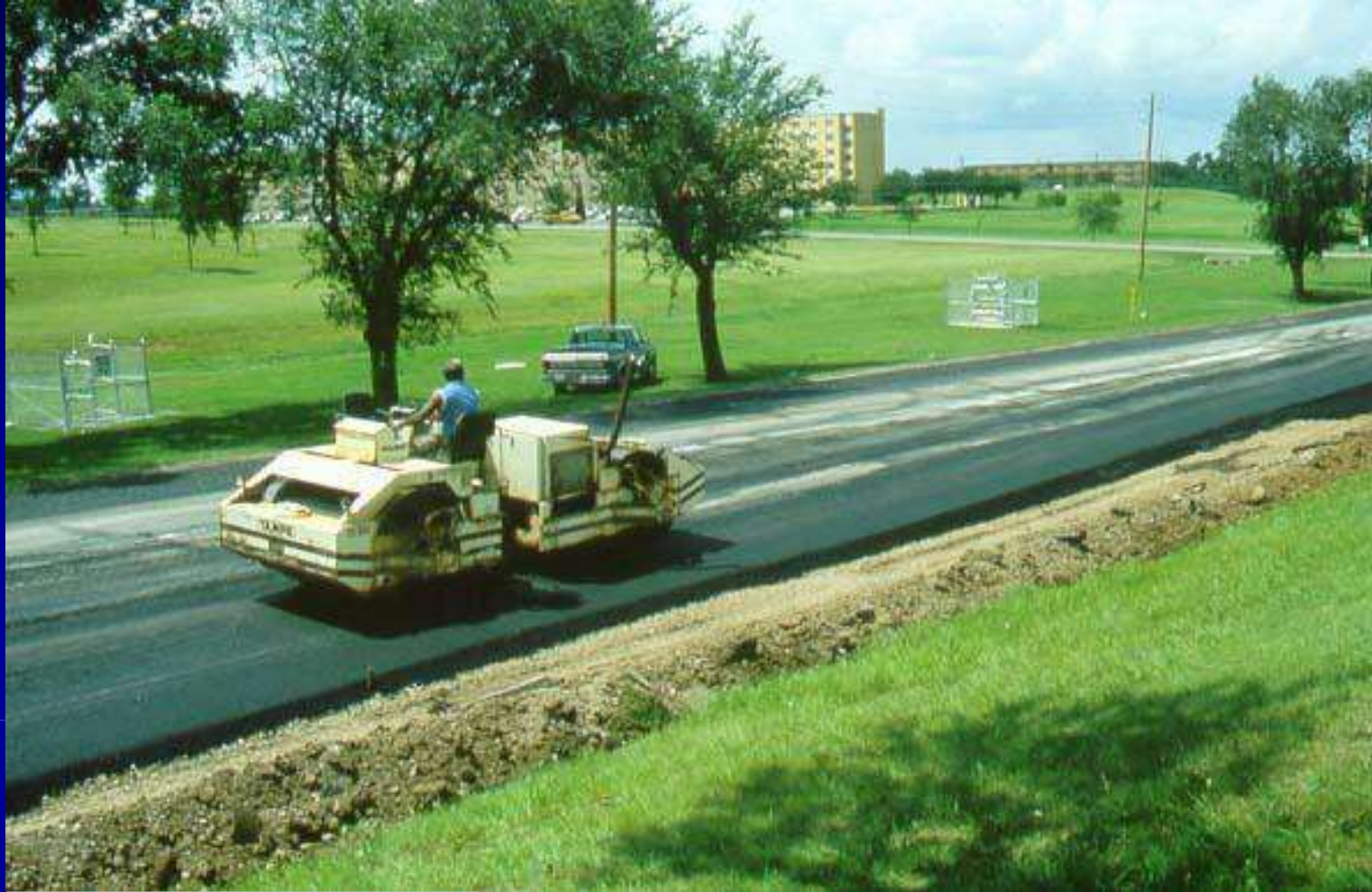
Patch Repaired Section
