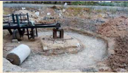
Compacted Subgrade by roller
