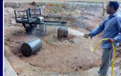
Preparation of sub-base with morrum soil
