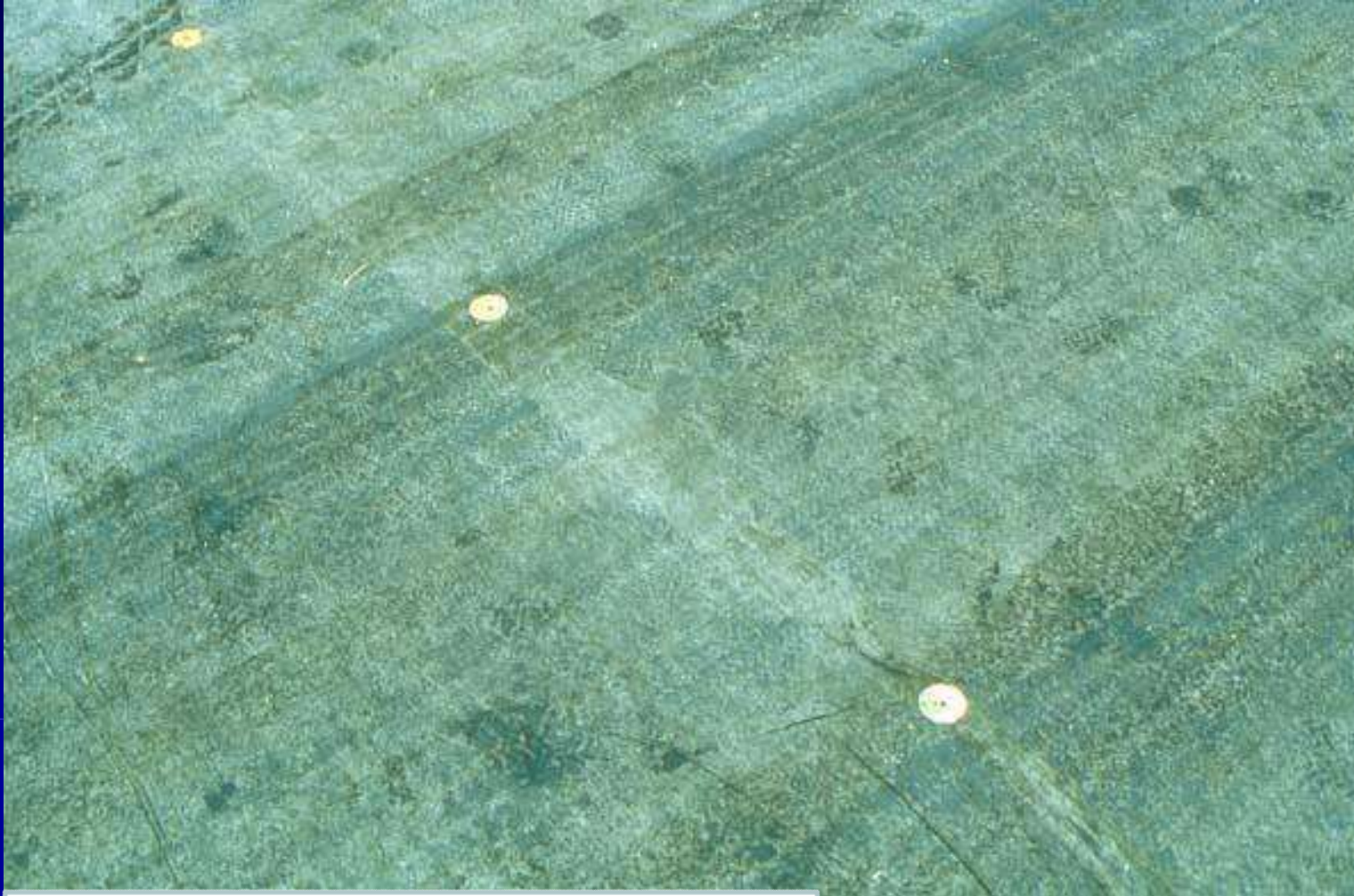
Transverse Joints Can Be Tacked In Place
