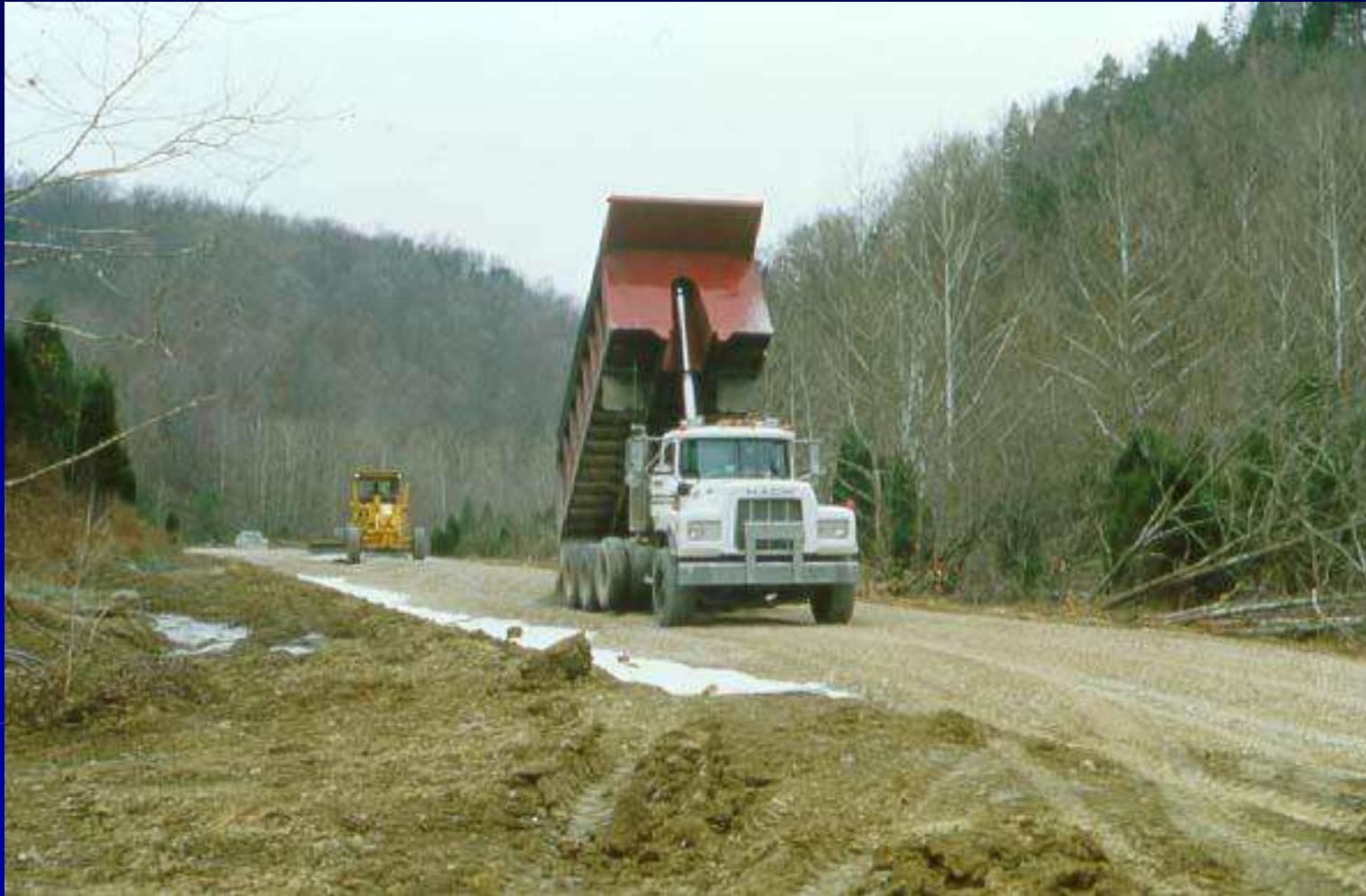
Rear Dumped Aggregate
