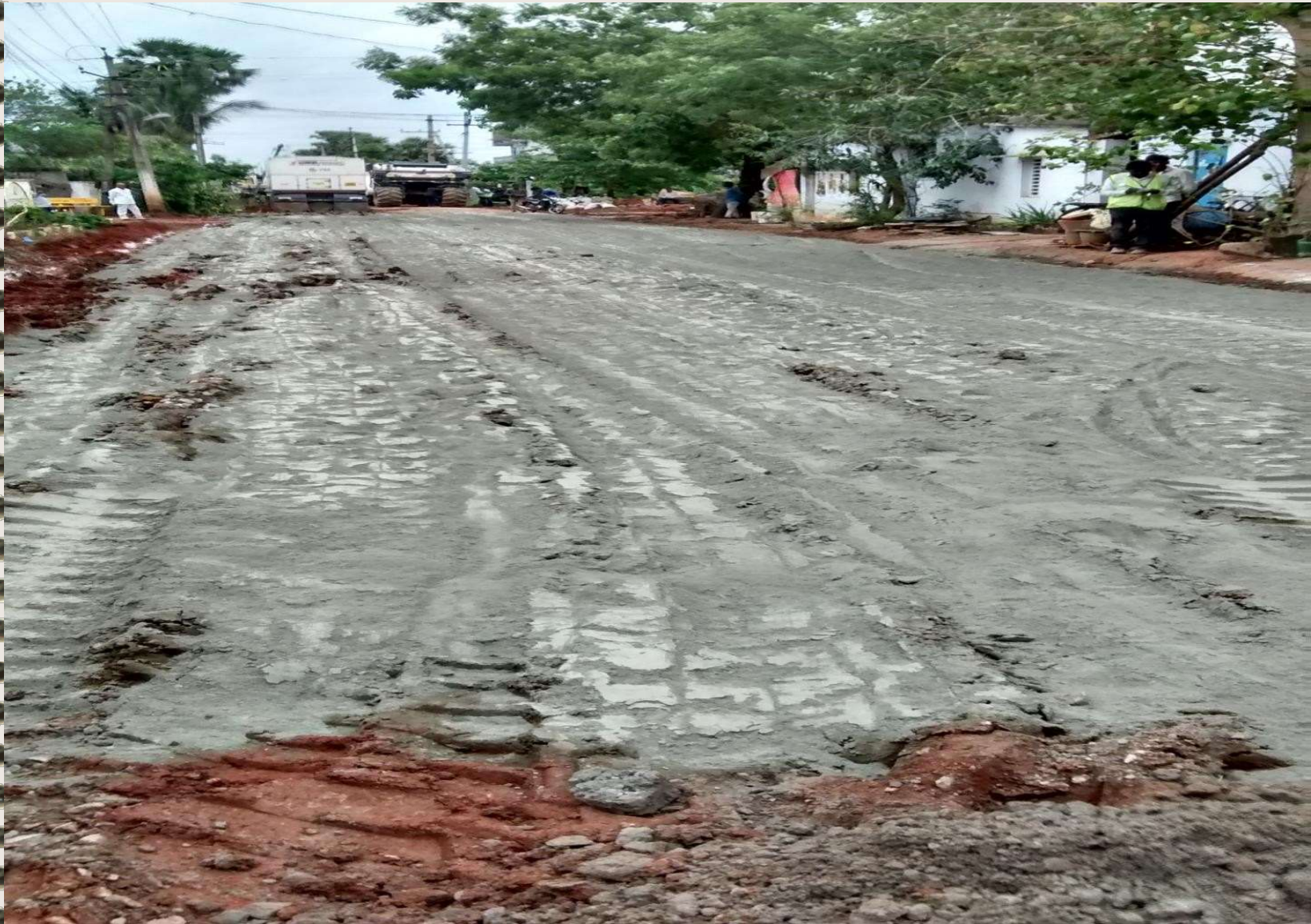
Spreading of Cement + Stabil © Road Compound, Vijayawada
