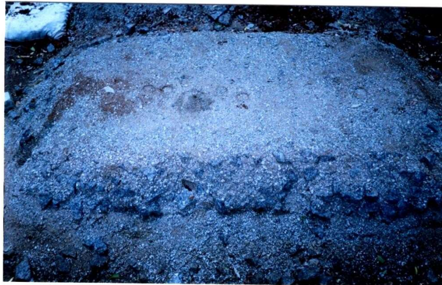
Plate 4.2 Untreated WBM stretch after monsoon rains
