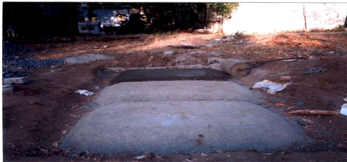
Plate 3.2 Completed WBM test stretches
