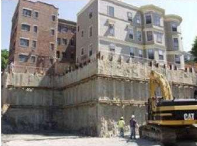
Top: Trench excavation railroad for an Alameda corridor project. Bottom: Structural cutoff wall during construction of new facility at Harvard University, Cambridge (Porbaha et al, 2005)
