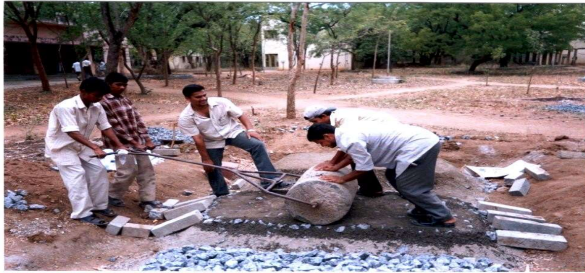
Plate 3.1 Rolling of Base course using 2 tonne stone roller
