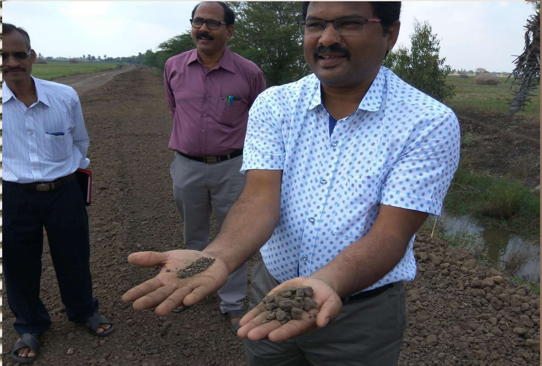
Attempt for Cement stabilisation Near Repalle, Guntur District
