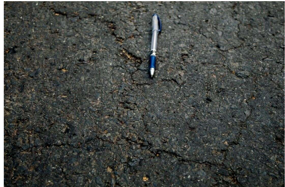
Cracking
