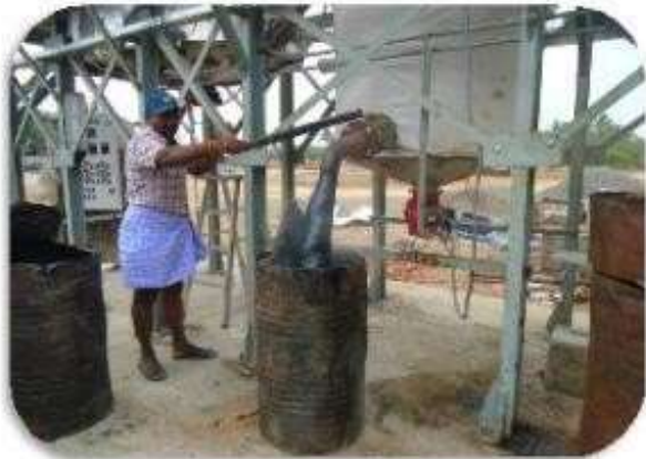
Filling & Despatching of CMR BITPLAST (Waste Plastic Impregnated Bitumen) to the Road site
