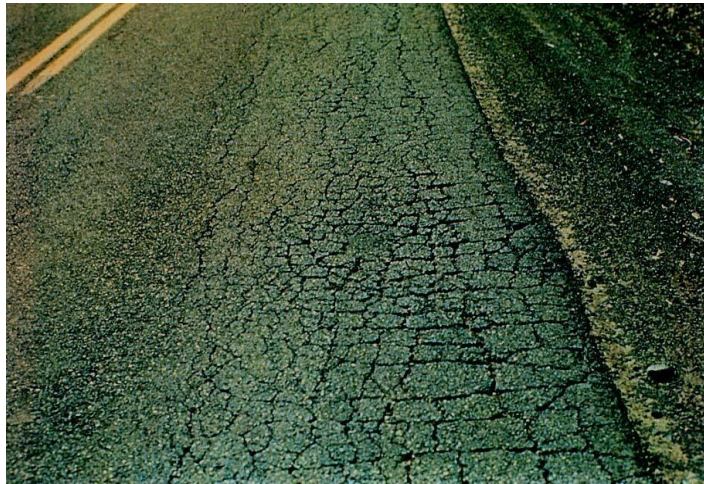
➤ Fatigue cracking
