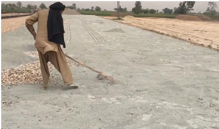
Packing/brooming of screening materials into the 46 voids of coarse aggregates
