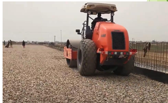
Compacting coarse aggregates using a static/vibratory roller
