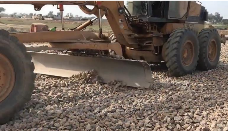
Spreading of aggregates using a grader
