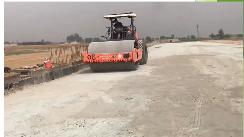
Applying vibration in-order to ensure packing of screening into coarse aggregates
