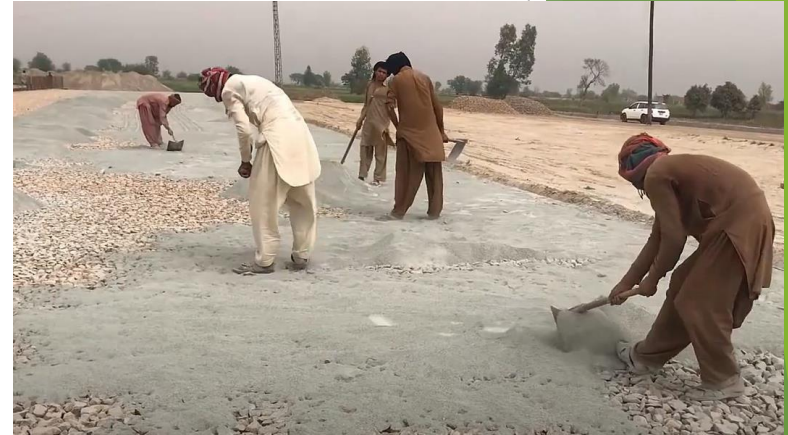
Spreading of screening materials
