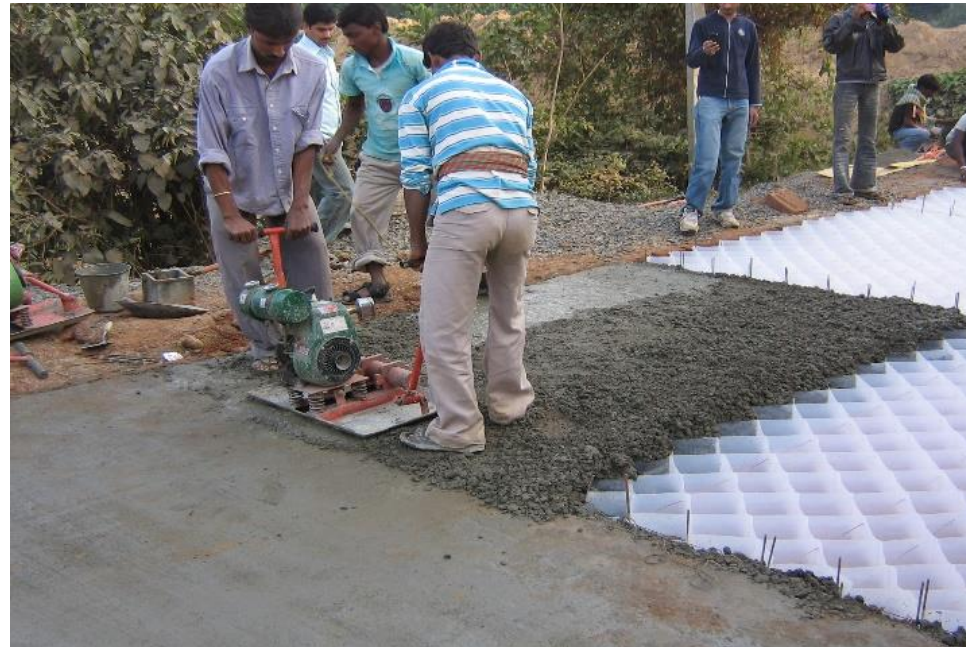
Cell-filled concrete block pavement
