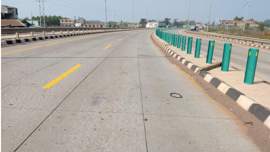
Short-panel concrete pavement on NH-18
