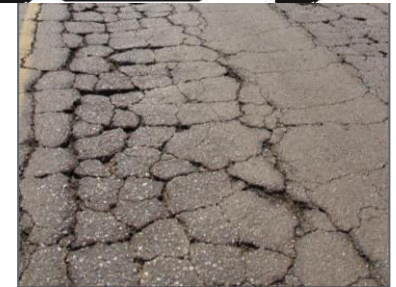
Cracked asphalt
