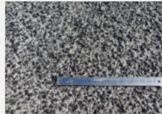
Single seal with emulsion cover spray and sand blinding
