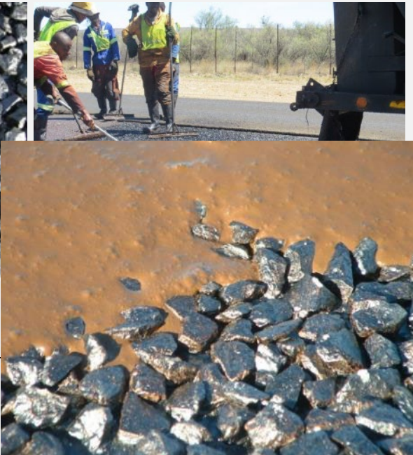
Hand application of slurry
