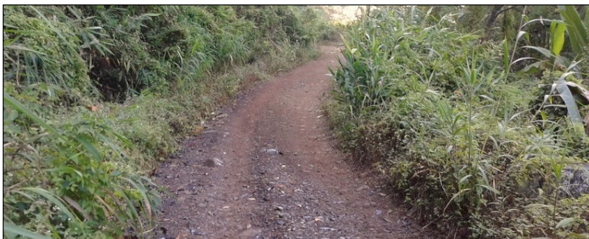
Fig 6.6: Rural road in hilly terrain in need of routine maintenance
