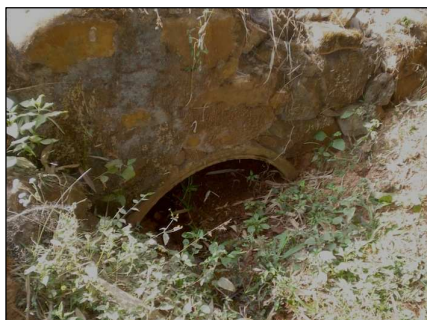
Fig 4.8: Blocked culvert
