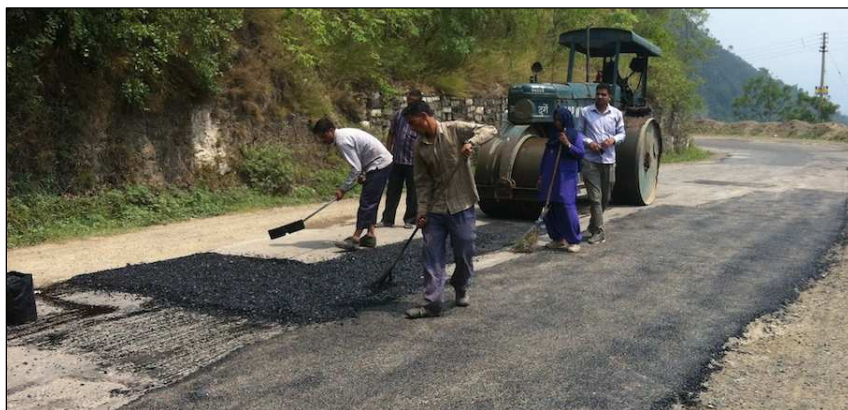
Fig 5.3: Maintenance by departmental labour in Himachal Pradesh
