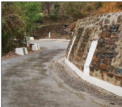
Fig 3.7: Retaining wall on a PMGSY road in Himachal Pradesh
