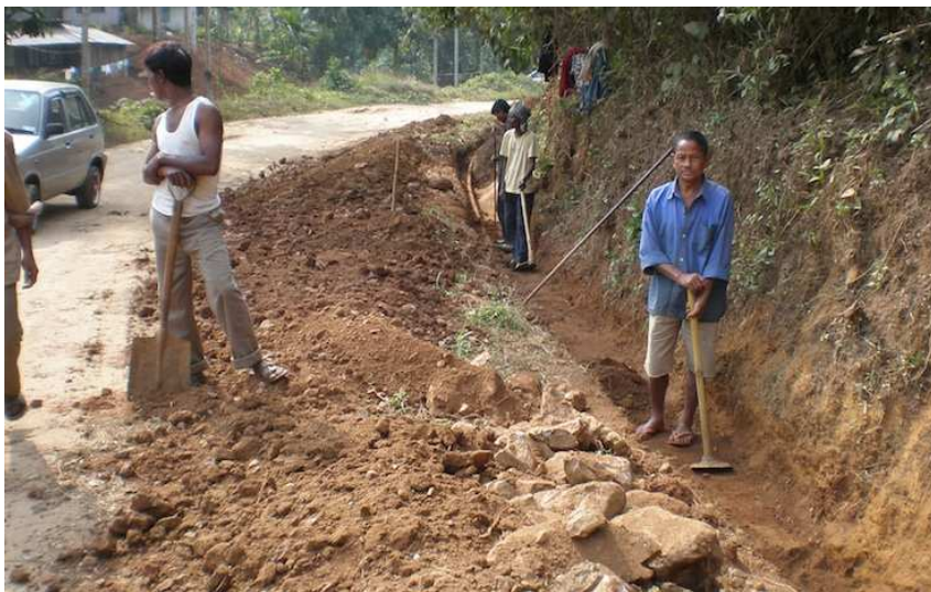
Fig 4.4: Excavating side drains, Meghalaya
