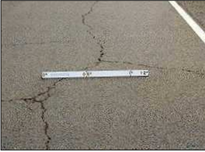
Fig 4.17: Large cracks
