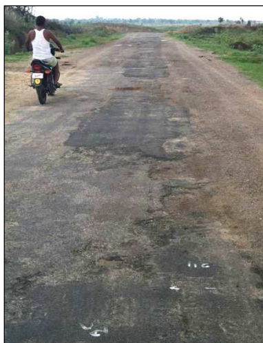
Fig 1.2: Road surface showing a history of routine maintenance, now due for resealing.
