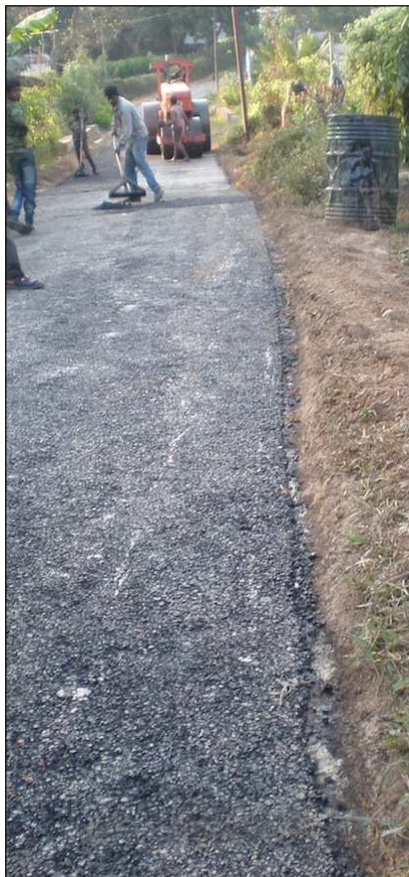
Fig 4.21: Resealing works in Meghalaya
