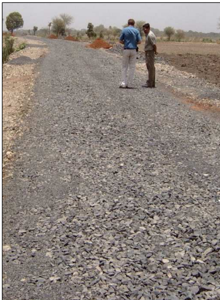
Fig 3.8: Good angular stone aggregate
