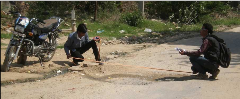
Fig 6.2: Assessing maintenance needs
