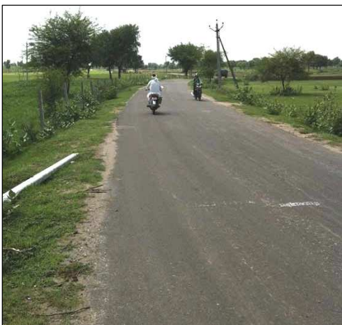
Fig 4.12: Good riding surface on PMGSY road, Rajasthan
