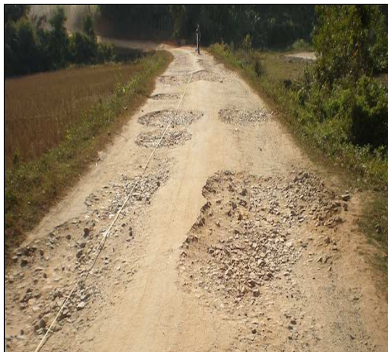
Fig 3.9: Catching up with long overdue maintenance
