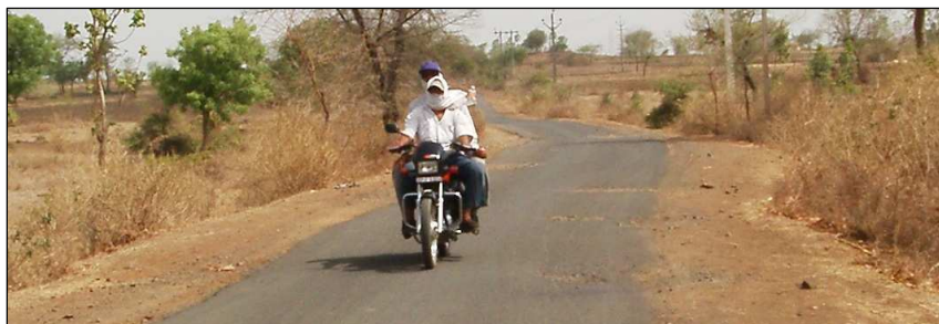
Fig 6.4: Road surface in need of patching works
