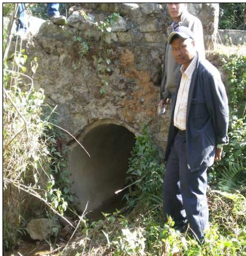
Fig 4.9: Culvert clear of debris
