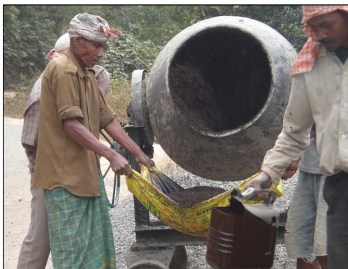
Fig 6.5: Mixing bitumen emulsion and aggregate for surfacing works
