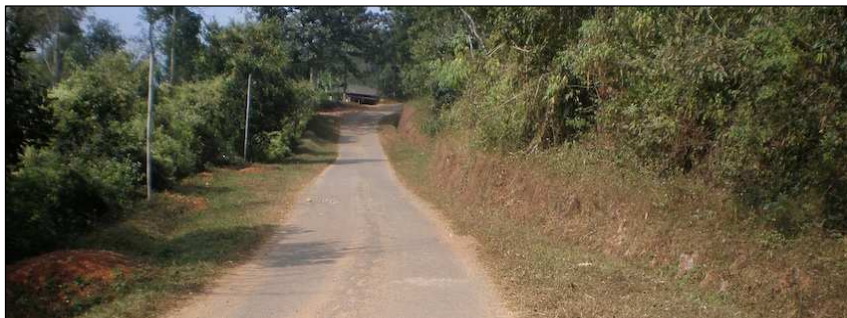
Fig 4.11: Vegetation neatly trimmed on shoulders and in drains
