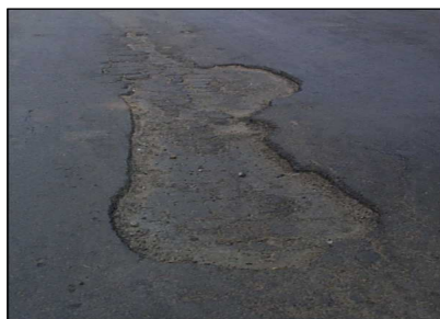
Fig 4.16: Delamination
