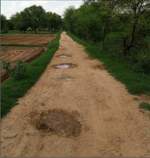
Fig 3.3: Village road built with inputs from MGNREGS
