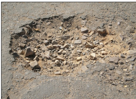
Fig 4.3: Progression to Pot-Hole
