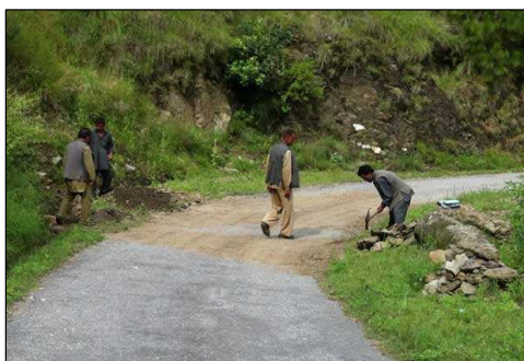
Fig 1.1: Routine maintenance of a culvert
