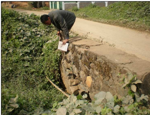
Fig 2.6: Regular inspections form the basis for effective maintenance management
