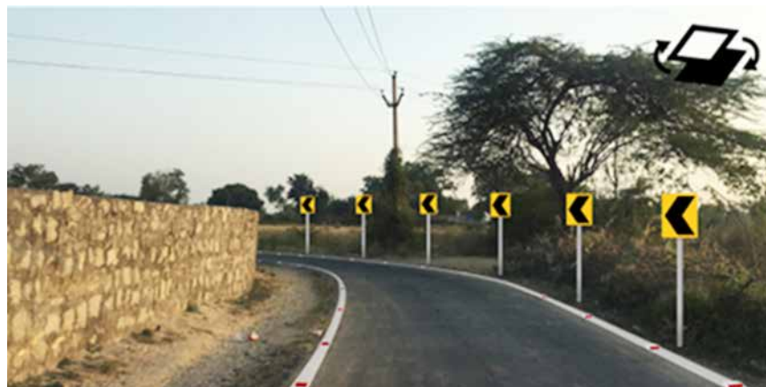
Fig. 14.13: Chevron Signs at Sharp Bend
