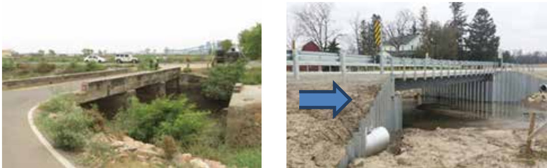
Fig. 14.8: Crash Barriers on approaches to Bridges
