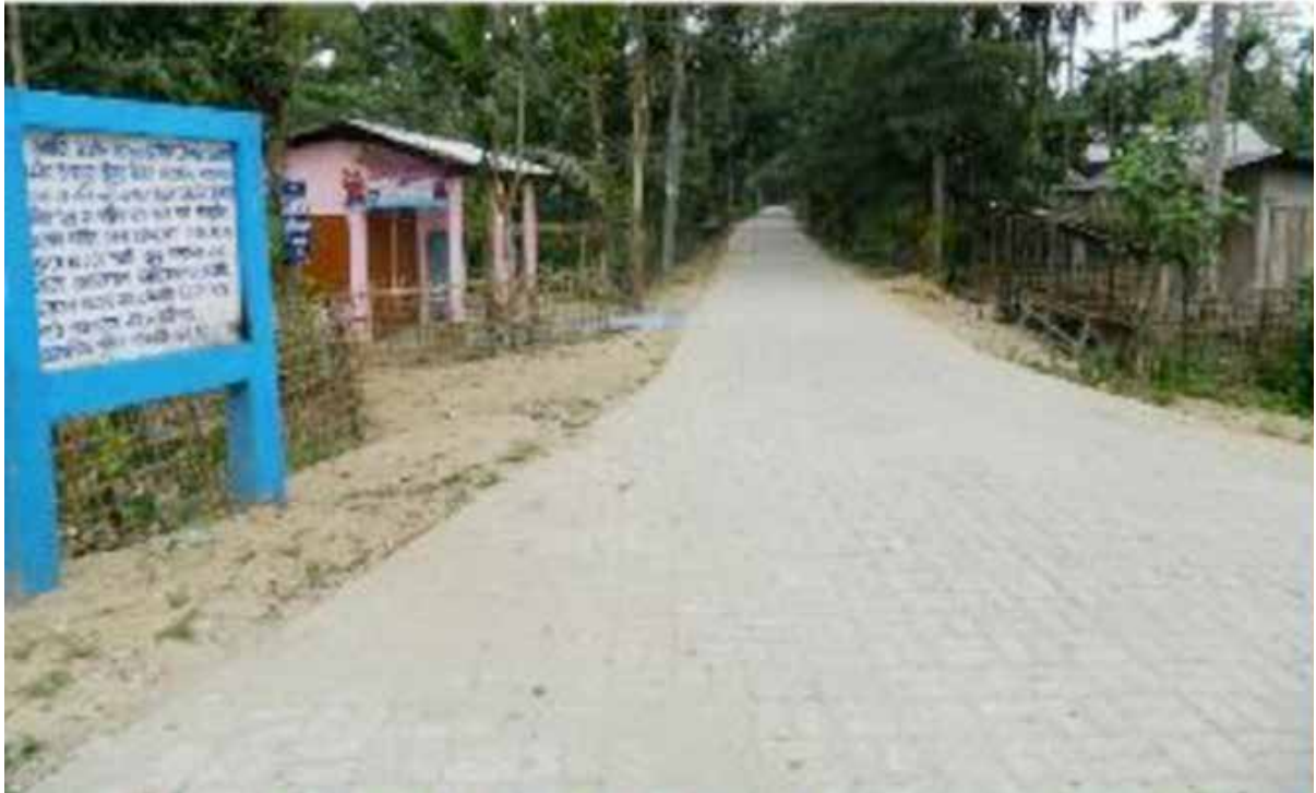
Fig. 14.15: Interlocking Concrete Blocks for Road Paving at Villages
