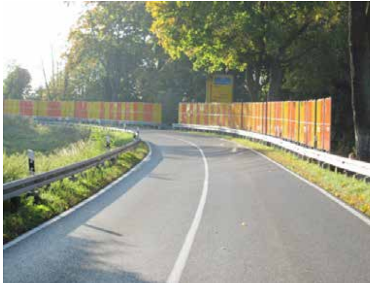
Fig. 14.14: Suggestive Low Cost Measures for Delineating at Sharp Bend
