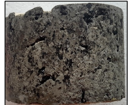
Full Depth grouting
