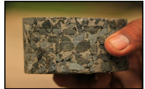
Side View of core taken from pavement showing full depth grout
