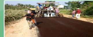
BitChem Coldmix Road in Nellore, Andhra Pradesh in 2018
