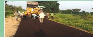
BitChem Coldmix Road at Mahabubabad, Telangana
