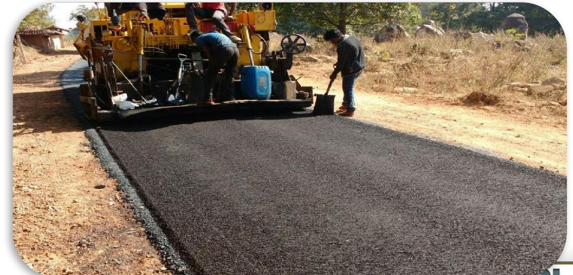
BitChem Coldmix Road at Raipur, Chattisgarh
