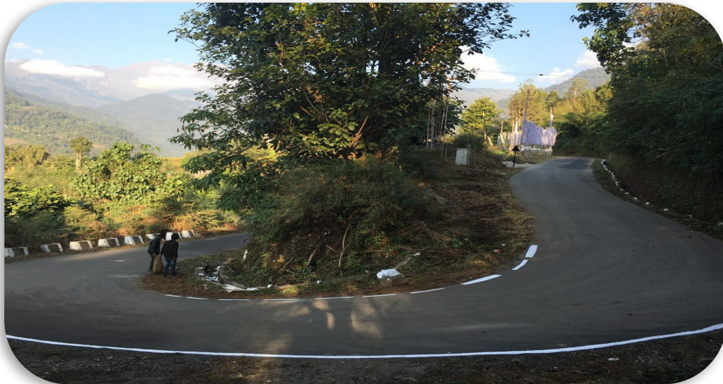
BitChem Cold mix Road at Sikkim
