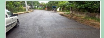
BitChem Coldmix Road at Chokladhara road, Jorhat 2013
