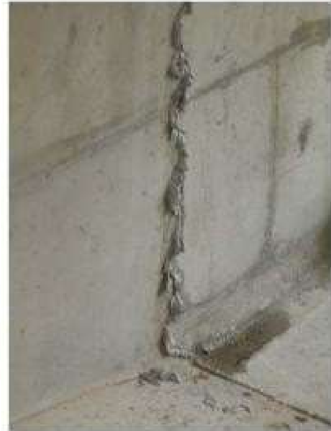
Appearance of Epoxy Glue after temporary prestress
