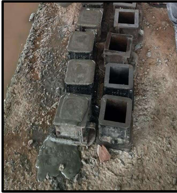
➤ Cube Casting of Grouting Mix
