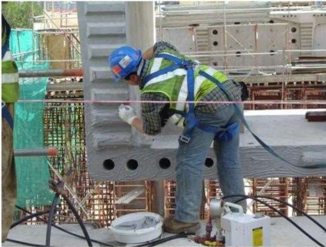
Hand application of Epoxy Glue
