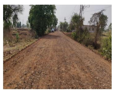
MUST: Compacted shoulders and proper drainage arrangement
