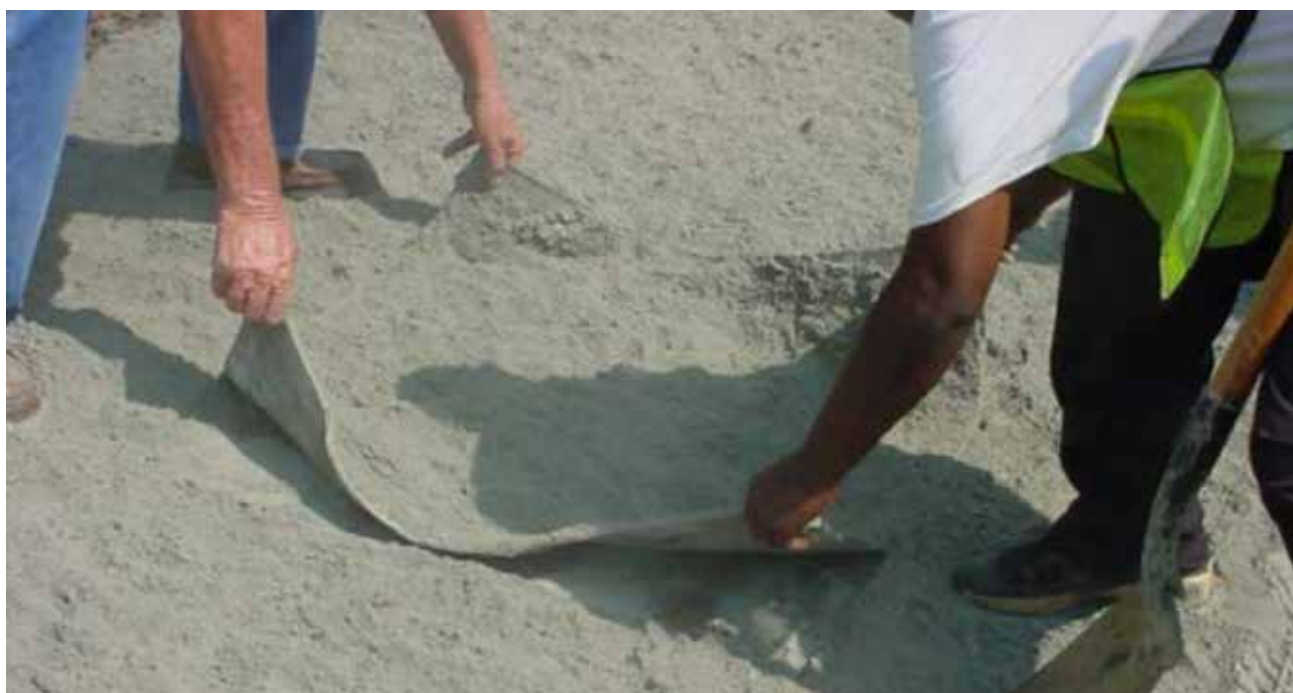
FIGURE 10: Cement application rate verification
