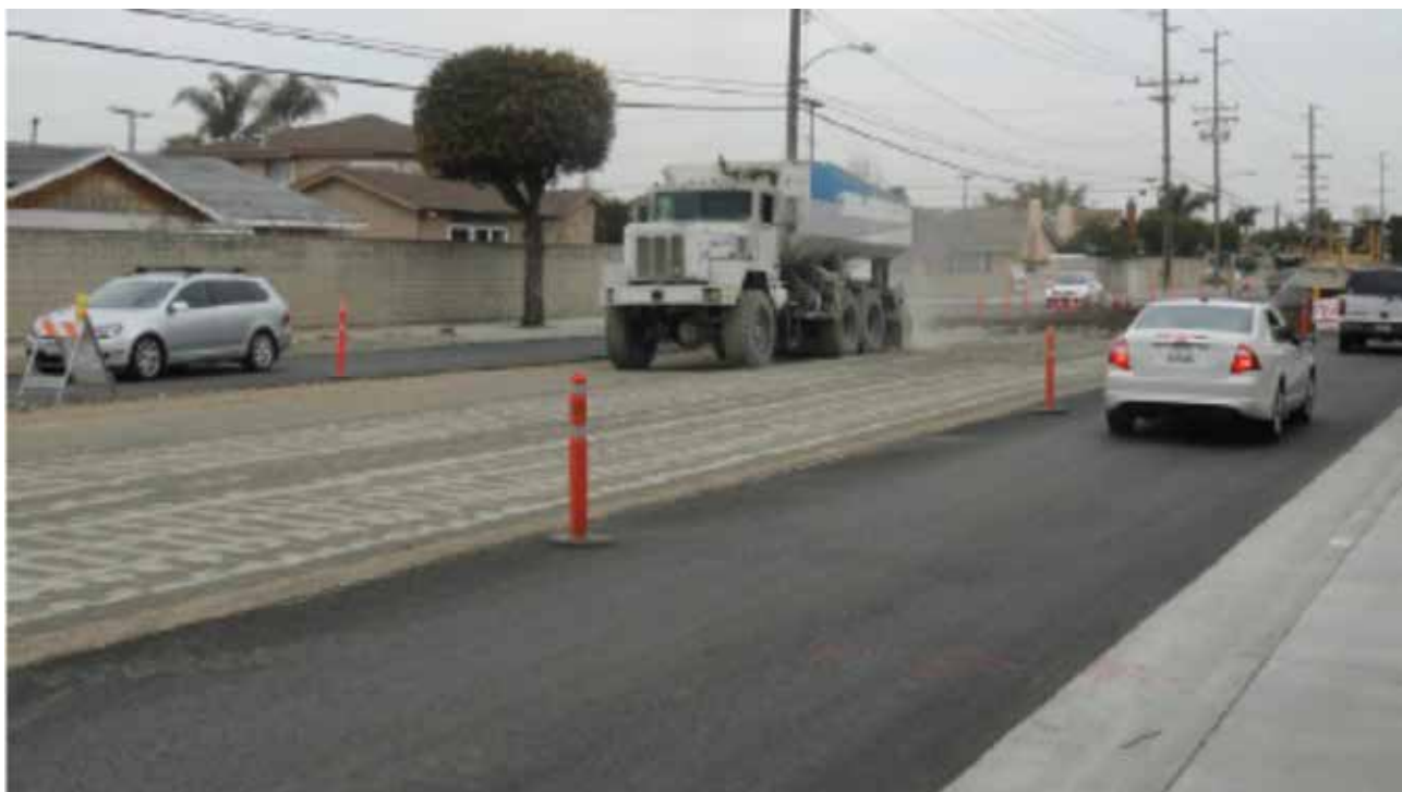
FIGURE 5: Application of dry cement powder to pulverized mix
