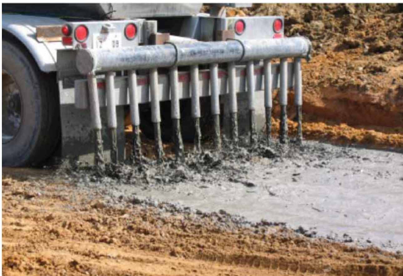
FIGURE 6: Application of cement slurry to pulverized mix
