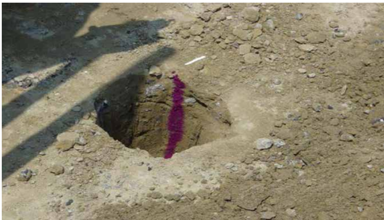
FIGURE 11: Phenolphthalein test at Site
