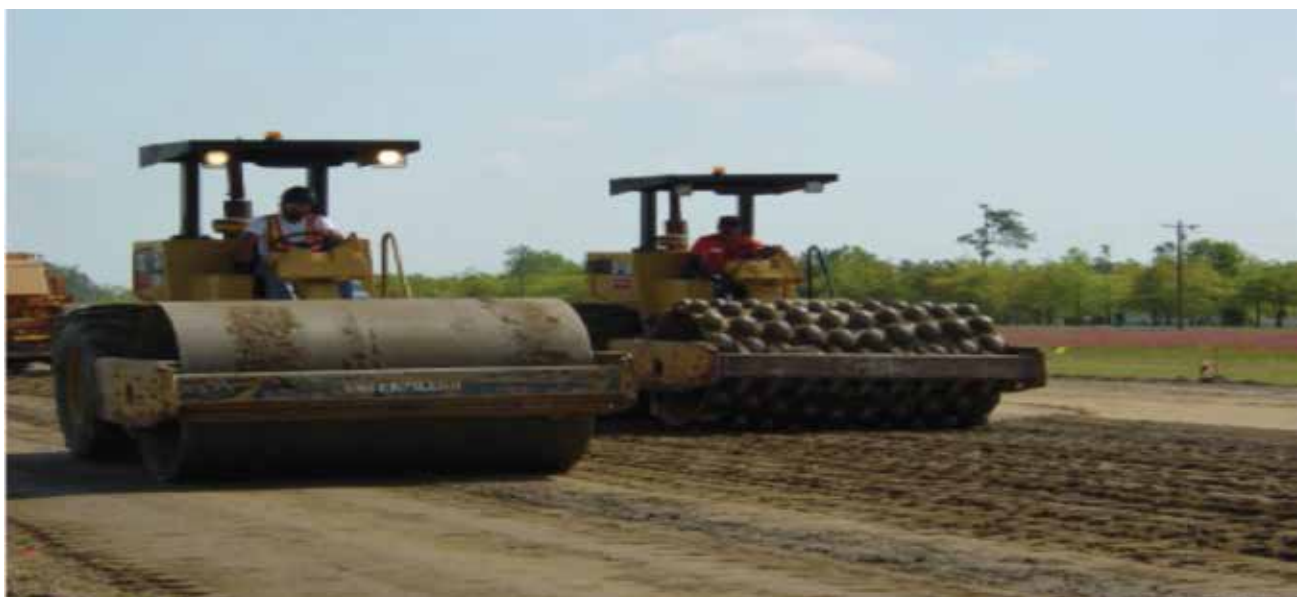
FIGURE 8: Final compaction of FDR base with a tamping roller (right) and Smooth Wheel Roller
