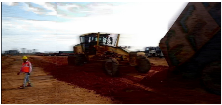
STEP 1: SOIL/EXISTING ROAD PROFILING
