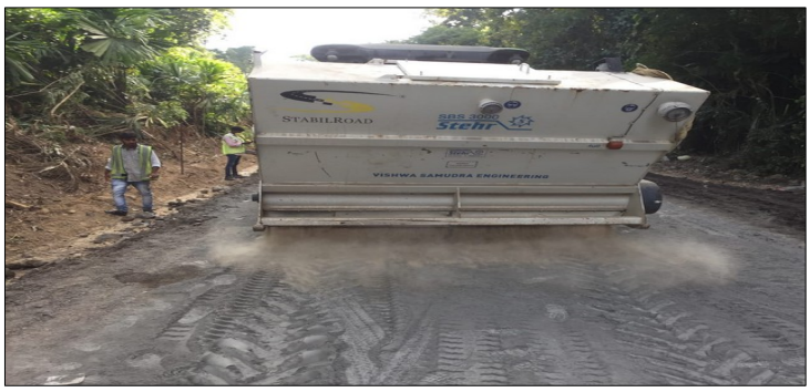
STEP 3: STABILROAD SPREADING
