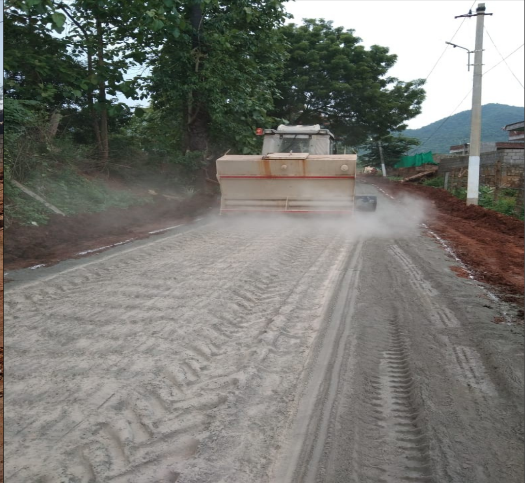
SPREADING OF STABILROAD ADDITIVE
