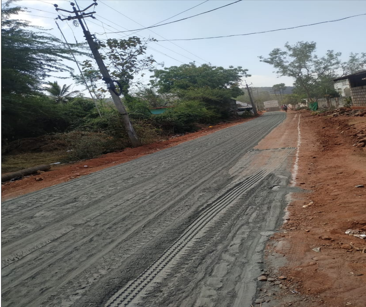
SPREADING OF CEMENT
