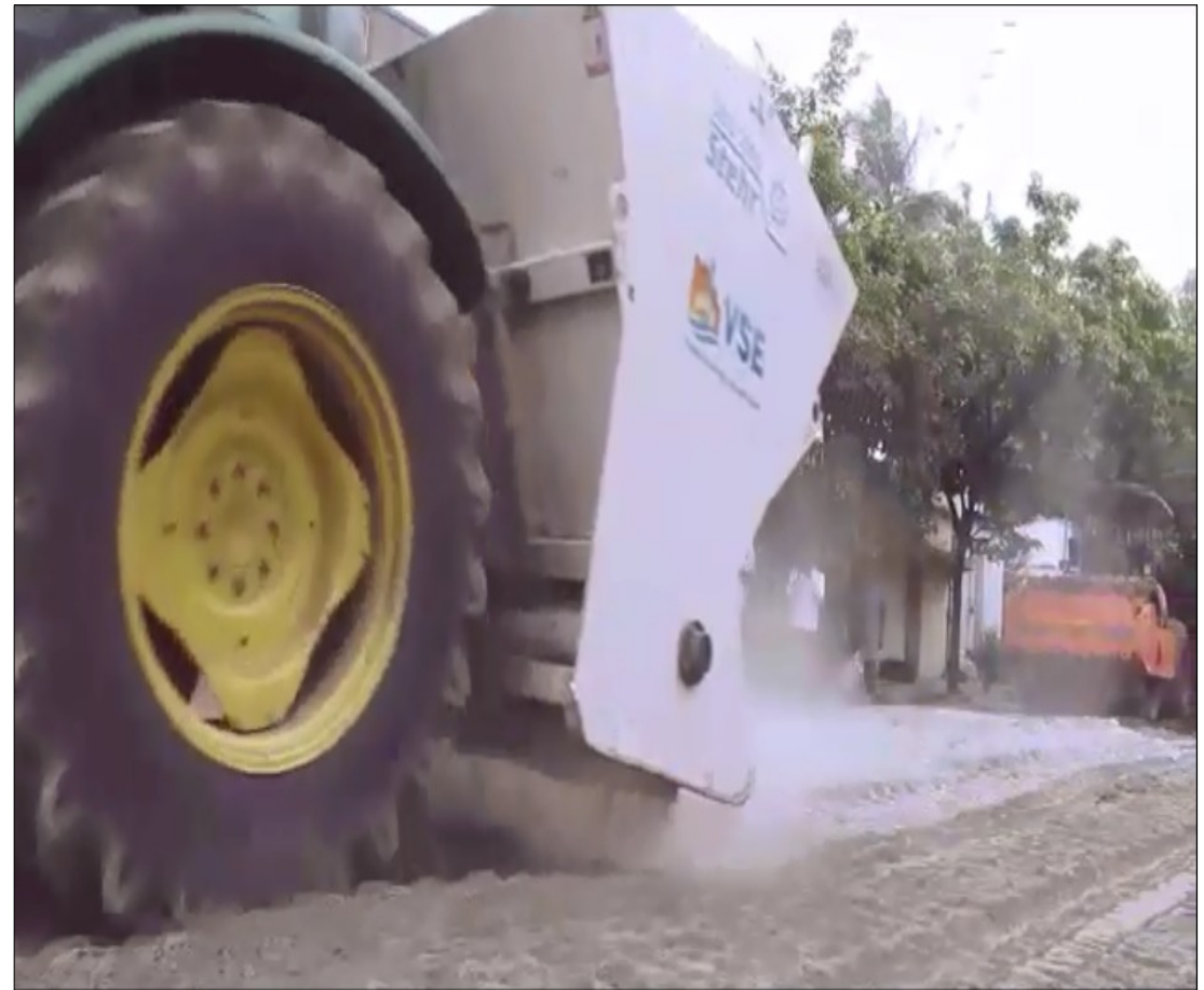
SPREADING OF STABILROAD ADDITIVE
