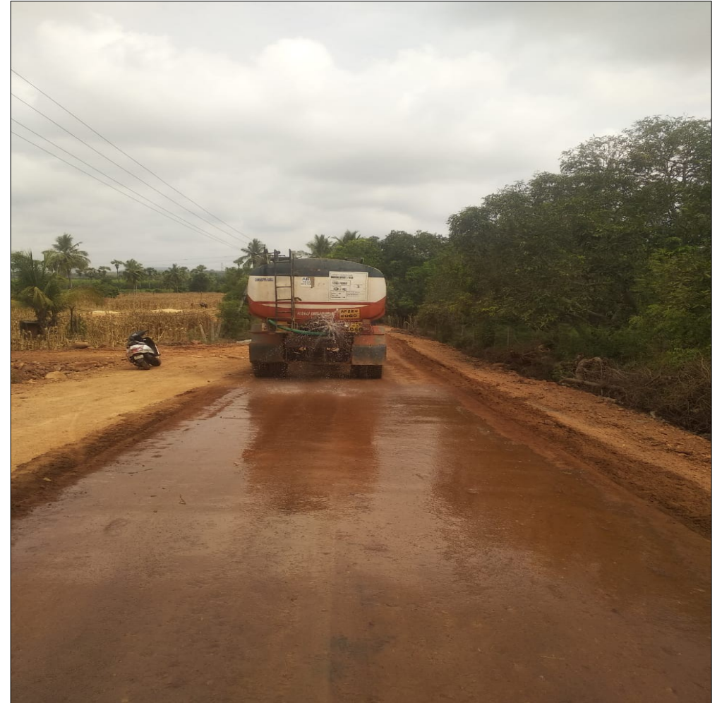
CURING AFTER FINAL COMPACTION
