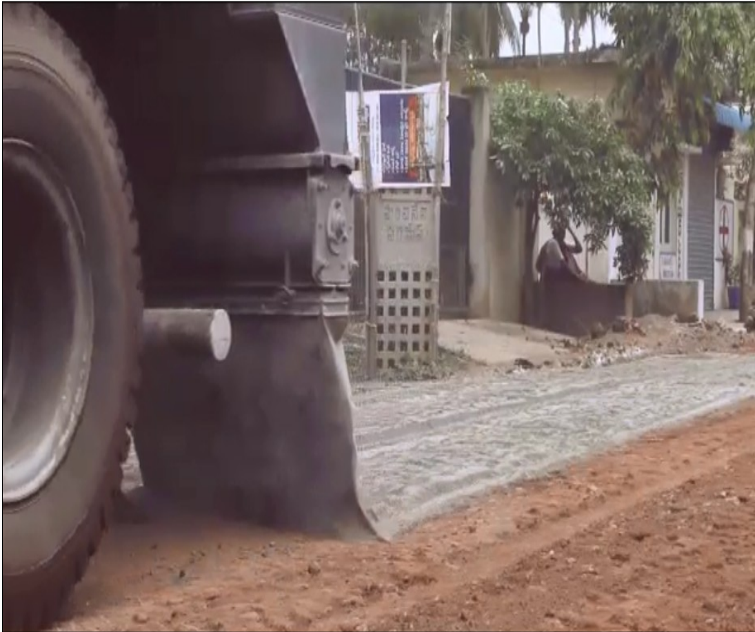
SPREADING OF CEMENT
