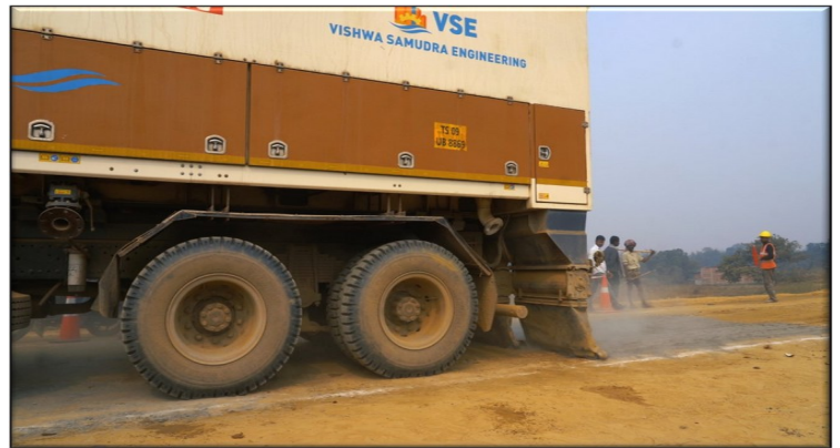
STEP 2: CEMENT SPREADING
