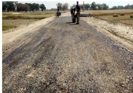
Spreading Prime & Tack Coat
