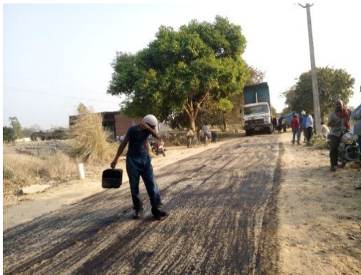
Spreading Prime & Tack Coat on JGT
