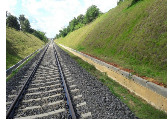
Slope Stabilized with Vegetative Cover
