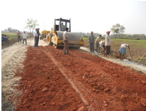
Sub-base spreading & roller compaction
