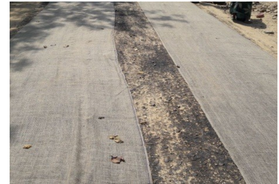
Laying of JGT
