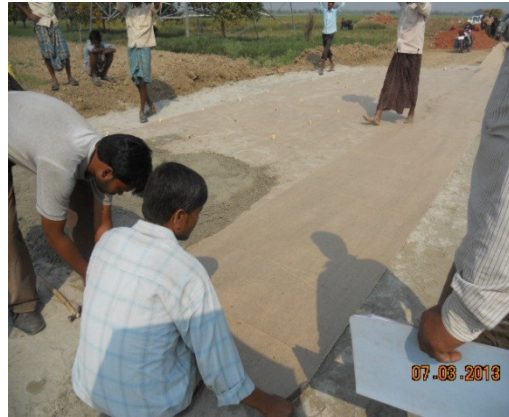
Laying of 724gsm woven JGT
