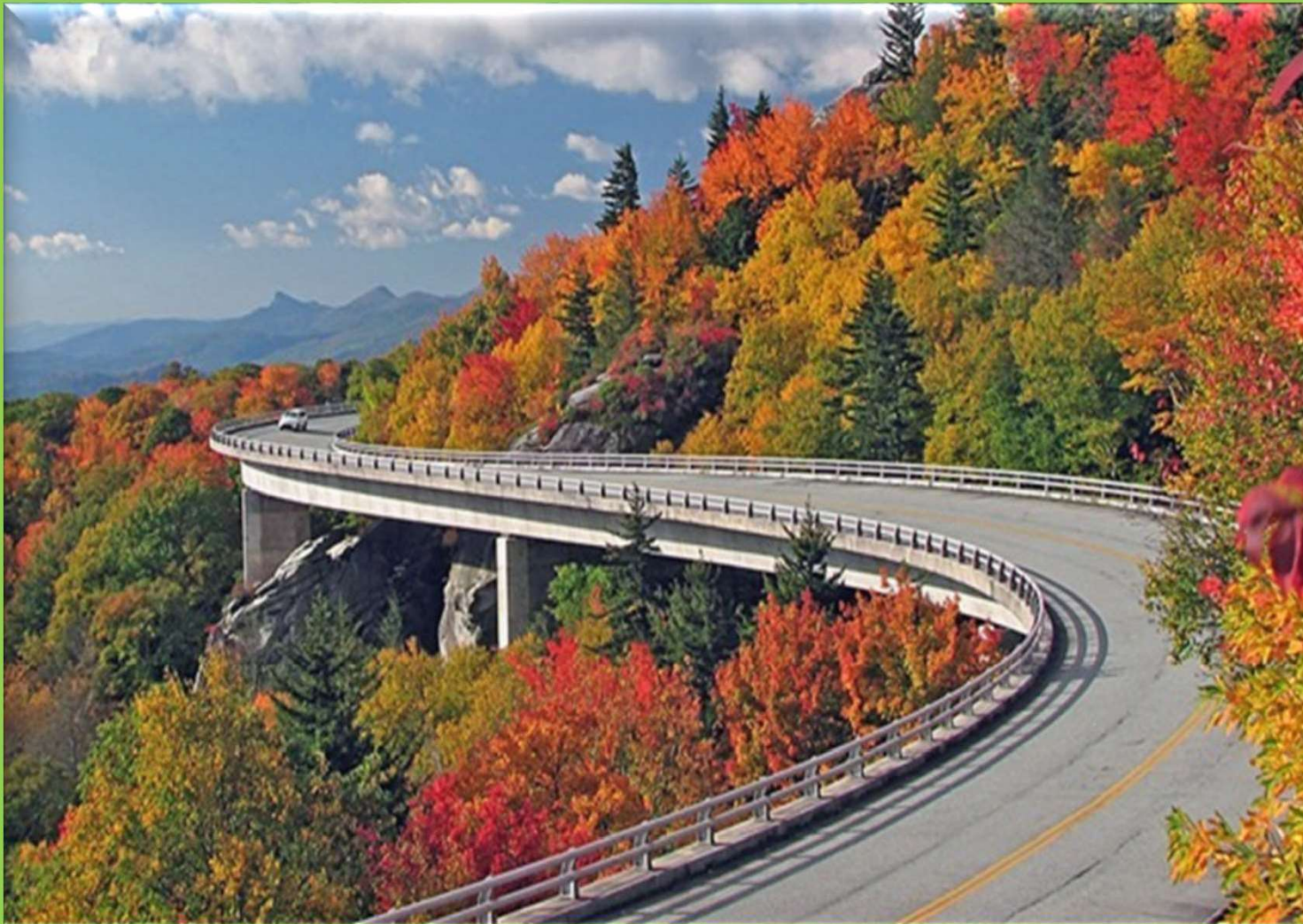
Linn Cove Viaduct, USA
