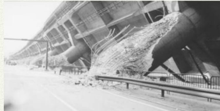
Higashi-Nada Viaduct collapse in 1995 Hyogo-Ken Nambu Earthquake, Jan 17, 1995.
