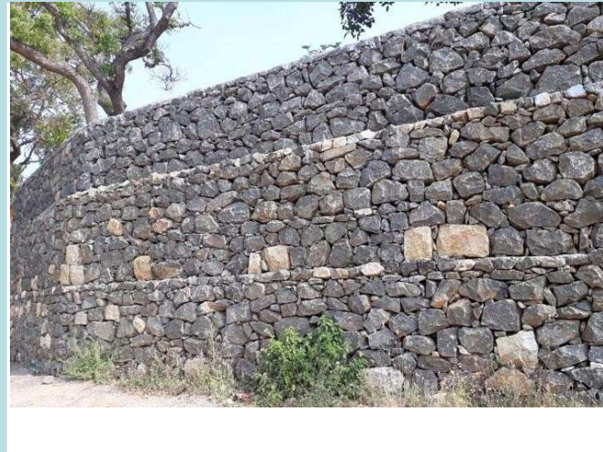
RR Masonry Retaining Walls
