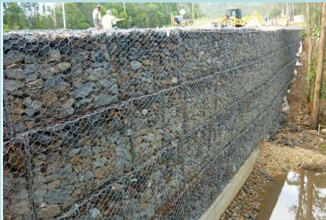
Gabion Retaining Walls
