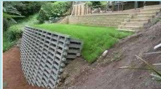
Crib Retaining Walls
