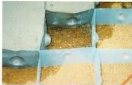
Dimpled formwork creates interlock between cells poured in situ (thin geocell formwork). (Hall & Hall 2007).
